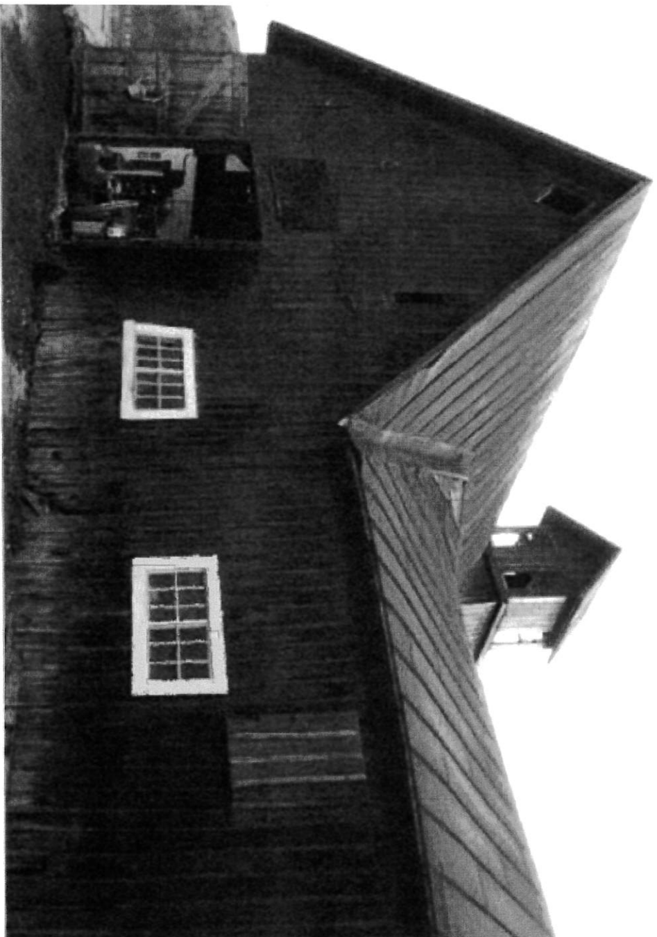
Fig. 2-35. Gable-front bank barn with board-and-batten siding and a cow stable ell at the right, circa 1870, Brookfield, Vermont.
