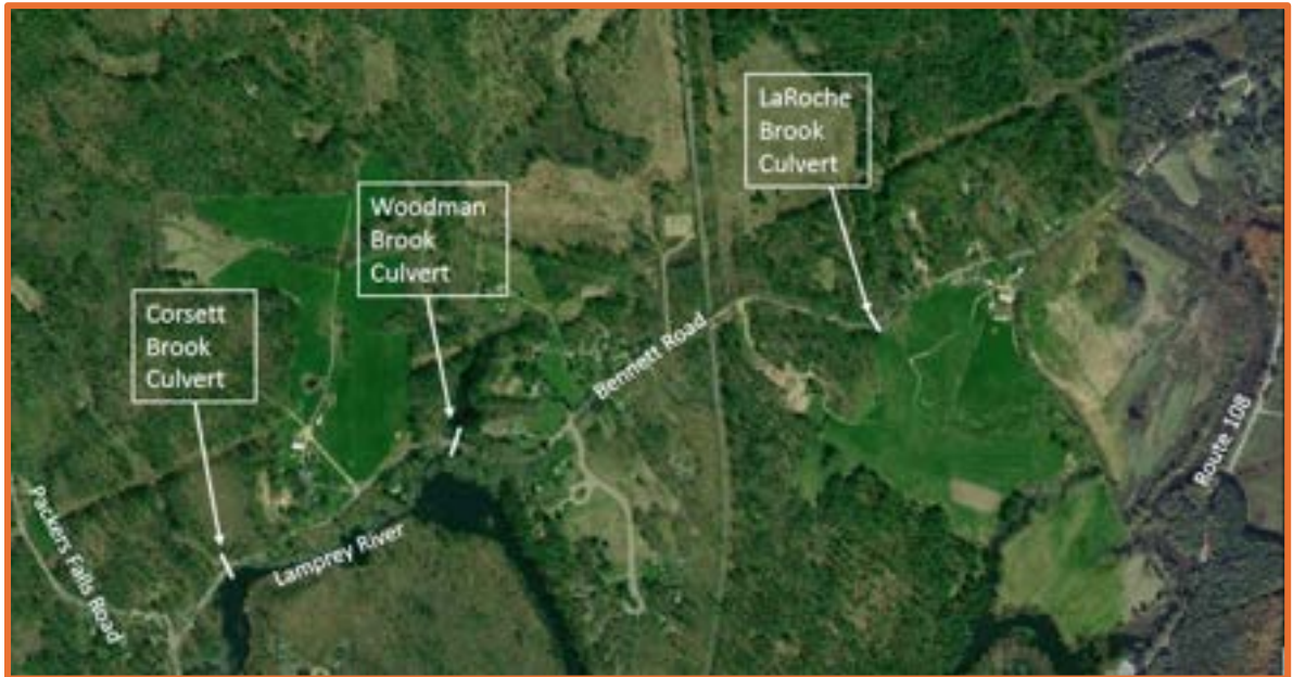
Bennett Road Culvert Locations
