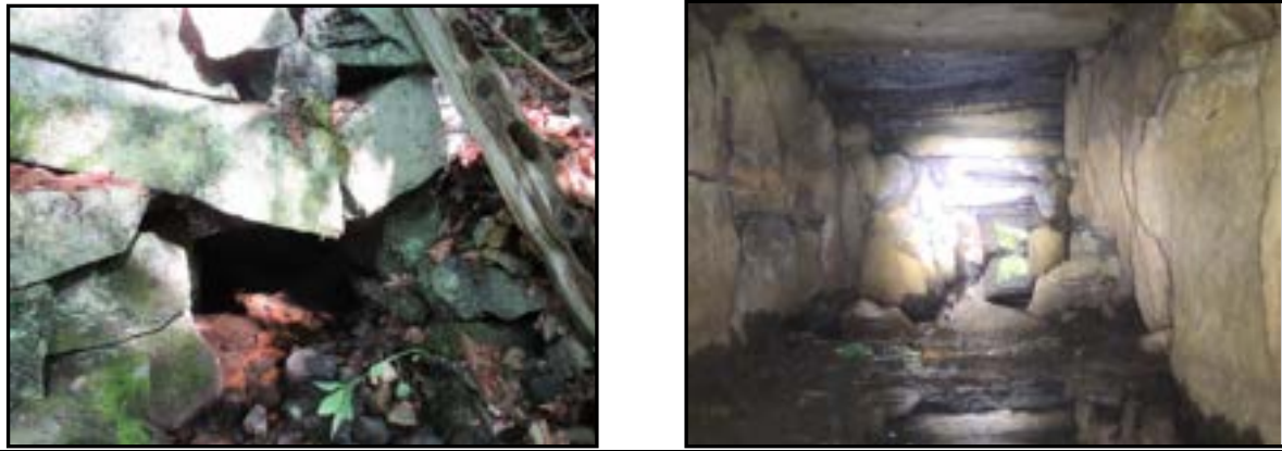
Snapped Stone at Outlet headwall – (Left) and Fallen Stones from Sidewall and Ceiling (Right) Littlehale Brook at Edgewood Road Stone Box Culvert
