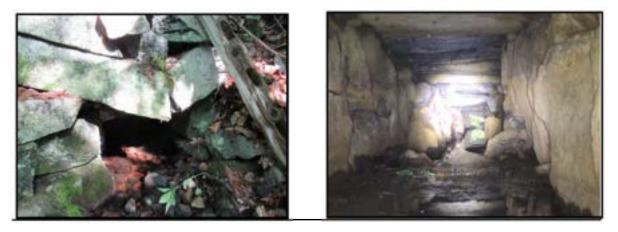
Snapped Stone at Outlet headwall – (Left) and Fallen Stones from Sidewall and Ceiling (Right) Littlehale Brook at Edgewood Road Stone Box Culvert
