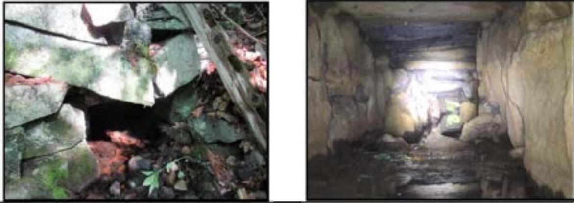
*Snapped Stone at Outlet headwall – (Left) and Fallen Stones from Sidewall and Ceiling (Right)
