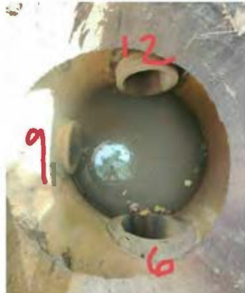
Photos above: Catch Basin structure on Schoolhouse Rd. with pipe locations.
