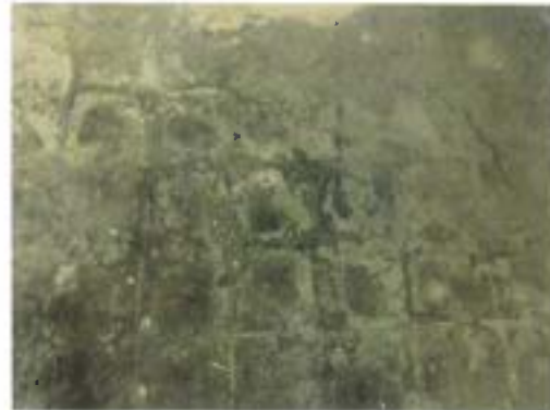
Figure 4: Detail of floor. Asbestos tiles were removed in 2010 because they were breaking up. They were not replaced.
