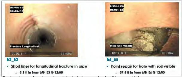
Photos above showing pipe defects to be repaired with sewer lining.
