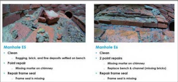
Photos above showing manhole defects to be repaired by manhole lining.
