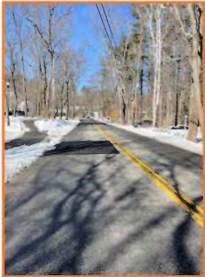
Emerson Road at Edgewood Road approach - watermain break trench patches alligator cracking, and raveling.
