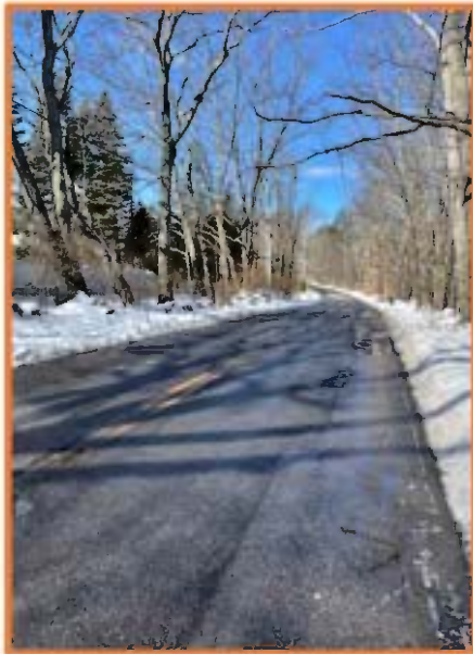
Emerson Road at western entrance to Littlehale Road - Severe Alligator Cracking and Rutting, Delamination and Base Failure
