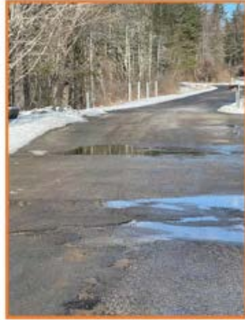
Durham Public Works Parking Lot showing pavement failures throughout
