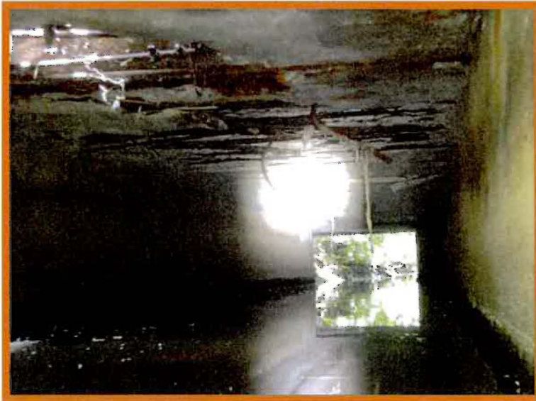
Madbury Road over Pettee Brook Inlet - Spalled Top Slab with Exposed Reinforcing Steel
