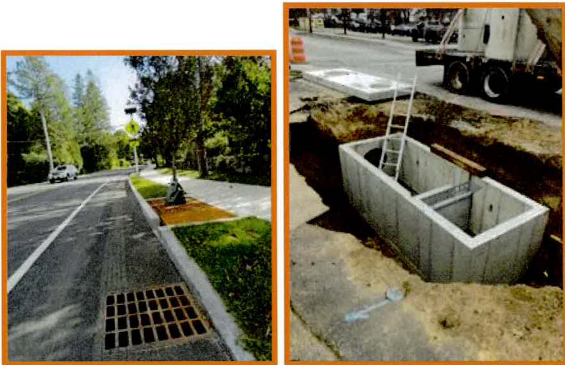
Pictured Above – Tree box filter (left) and Installation of Media Box Filter (right)
