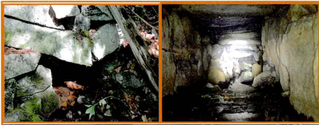
Snapped Stone at Outlet headwall – (Left) and Fallen Stones from Sidewall and Ceiling (Right) Littlehale Brook at Edgewood Road Stone Box Culvert
