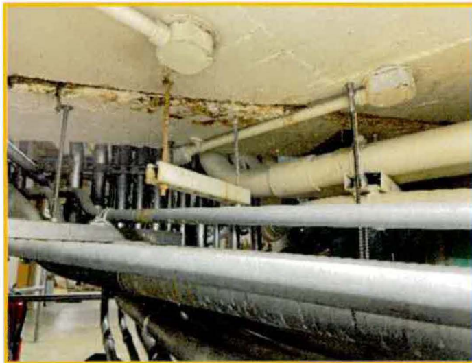
Pipe Gallery showing water intrusion at ceiling joint
