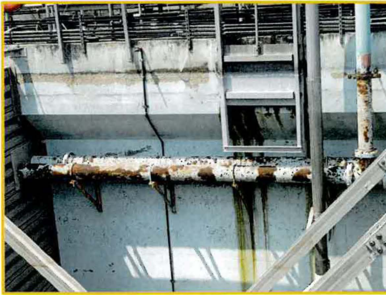
Aeration Tank showing corroded header and pipe supports
