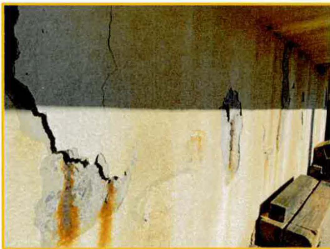
Control Building exhibiting concrete failure
