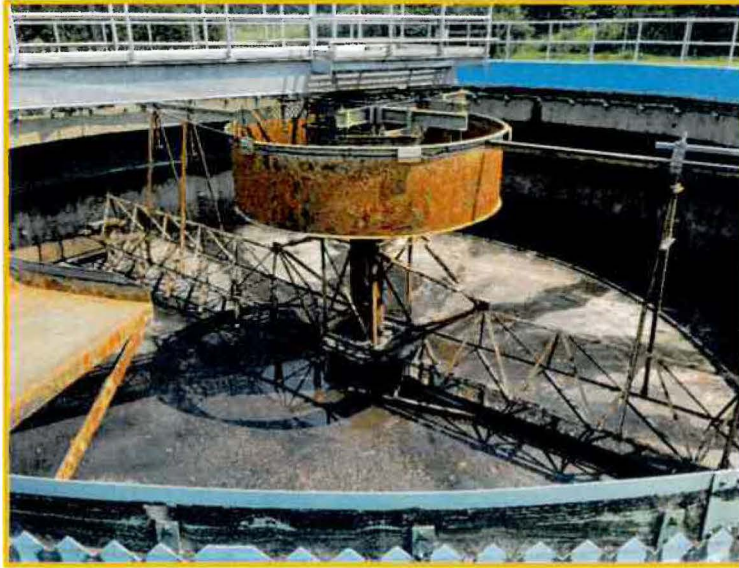
Secondary Clarifier with extensive corrosion. Note significant corroded/rusted material that fell off the mechanism shown on floor of clarifier
