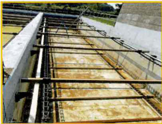
Primary Clarifier showing chain and flight collection system.
