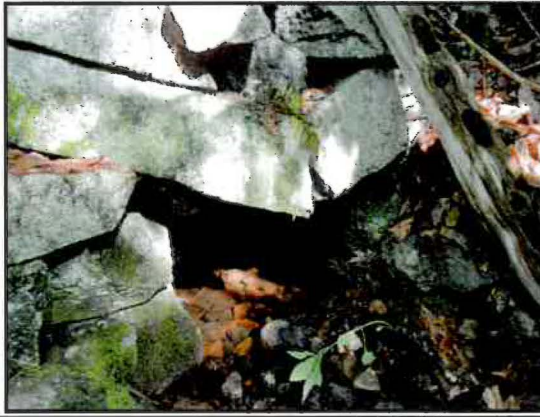
Snapped Stone at Outlet headwall – (Left) and Fallen Stones from Sidewall and Ceiling (Right) Littlehale Brook at Edgewood Road Stone Box Culvert
