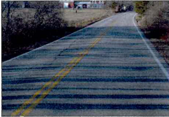
Back River Road - Alligator Cracking and Longitudinal Cracking
