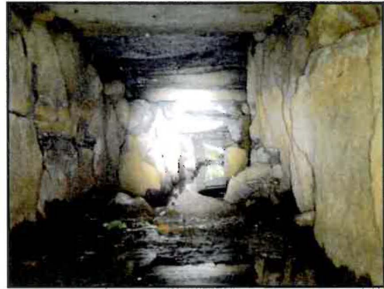
Snapped Stone at Outlet headwall – (Left) and Fallen Stones from Sidewall and Ceiling (Right) Littlehale Brook at Edgewood Road Stone Box Culvert
