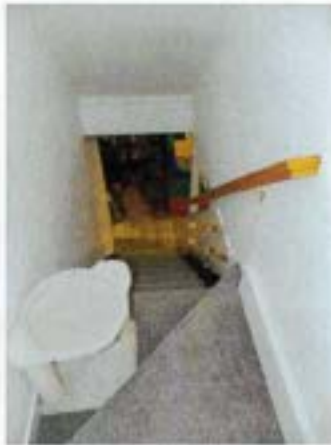
One of 2 Stairs to Basement
