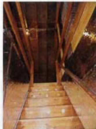
Stairs to Attic
