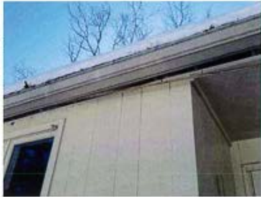
Exterior Trim — Deterioration
