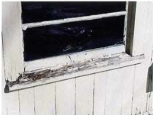
Garage Window Trim — Rot / Deterioration
