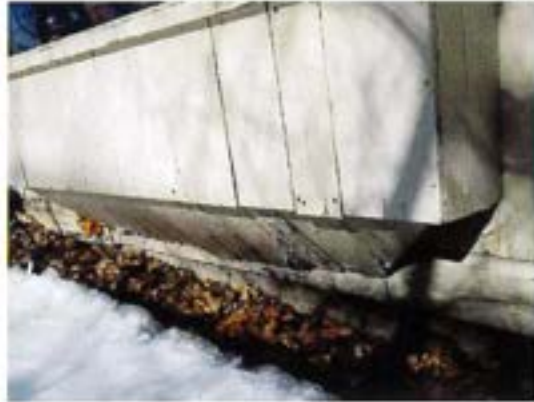
Exterior Siding — Peeling Paint / Deterioration
