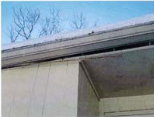
Exterior Trim — Deterioration
