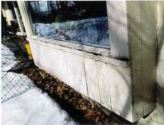
Exterior Siding — Peeling Paint / Deterioration
