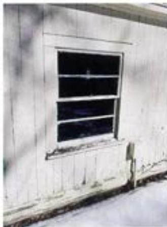
Garage Window Trim — Rot / Deterioration
