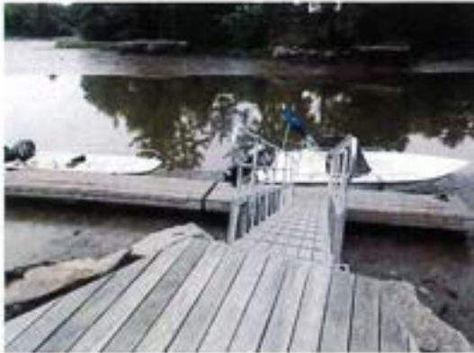
Former Dock Location - Structure Has Been Removed & No Longer Present (Owner-Provided Photo)
