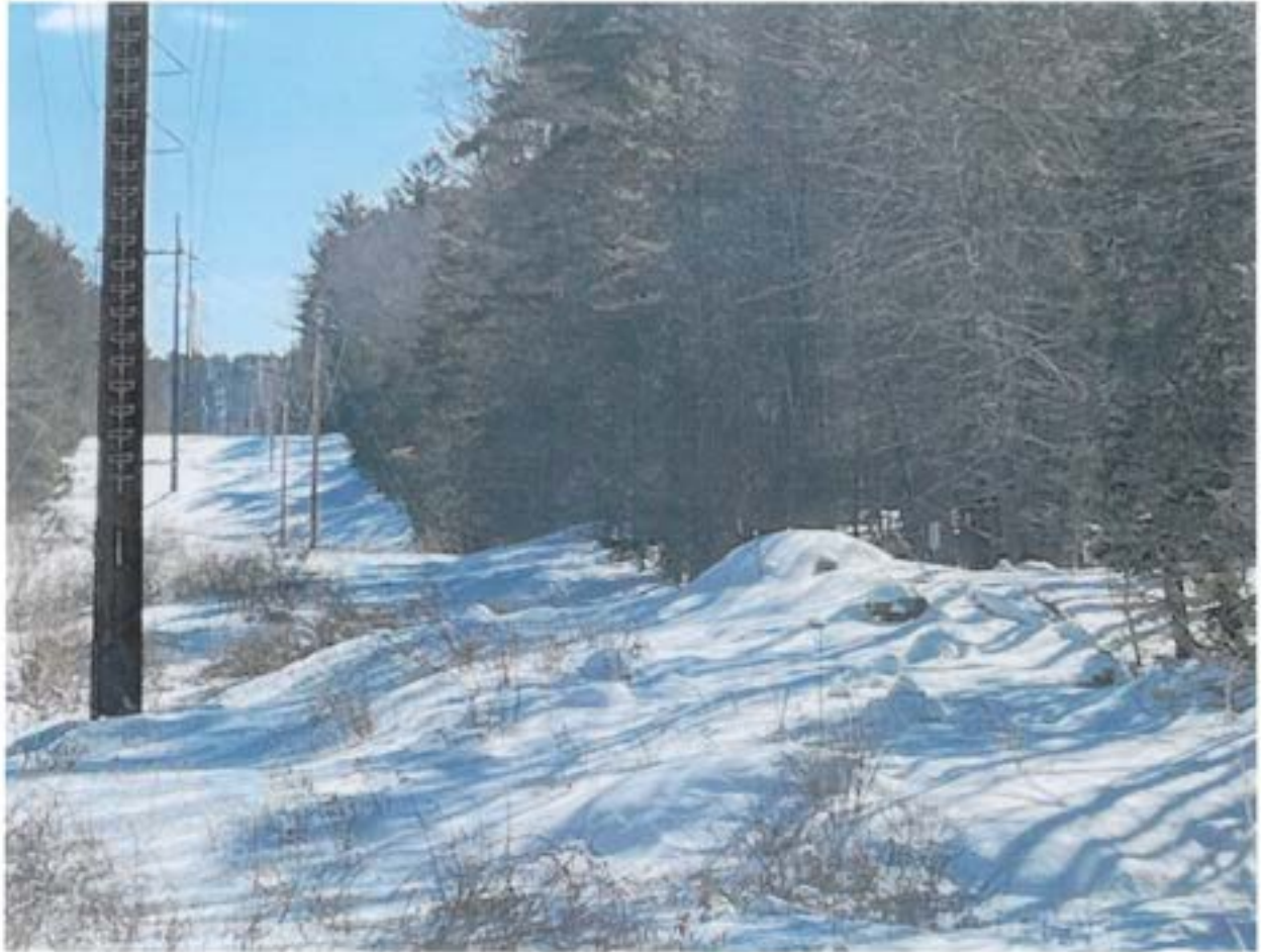
Hoard under power lines
