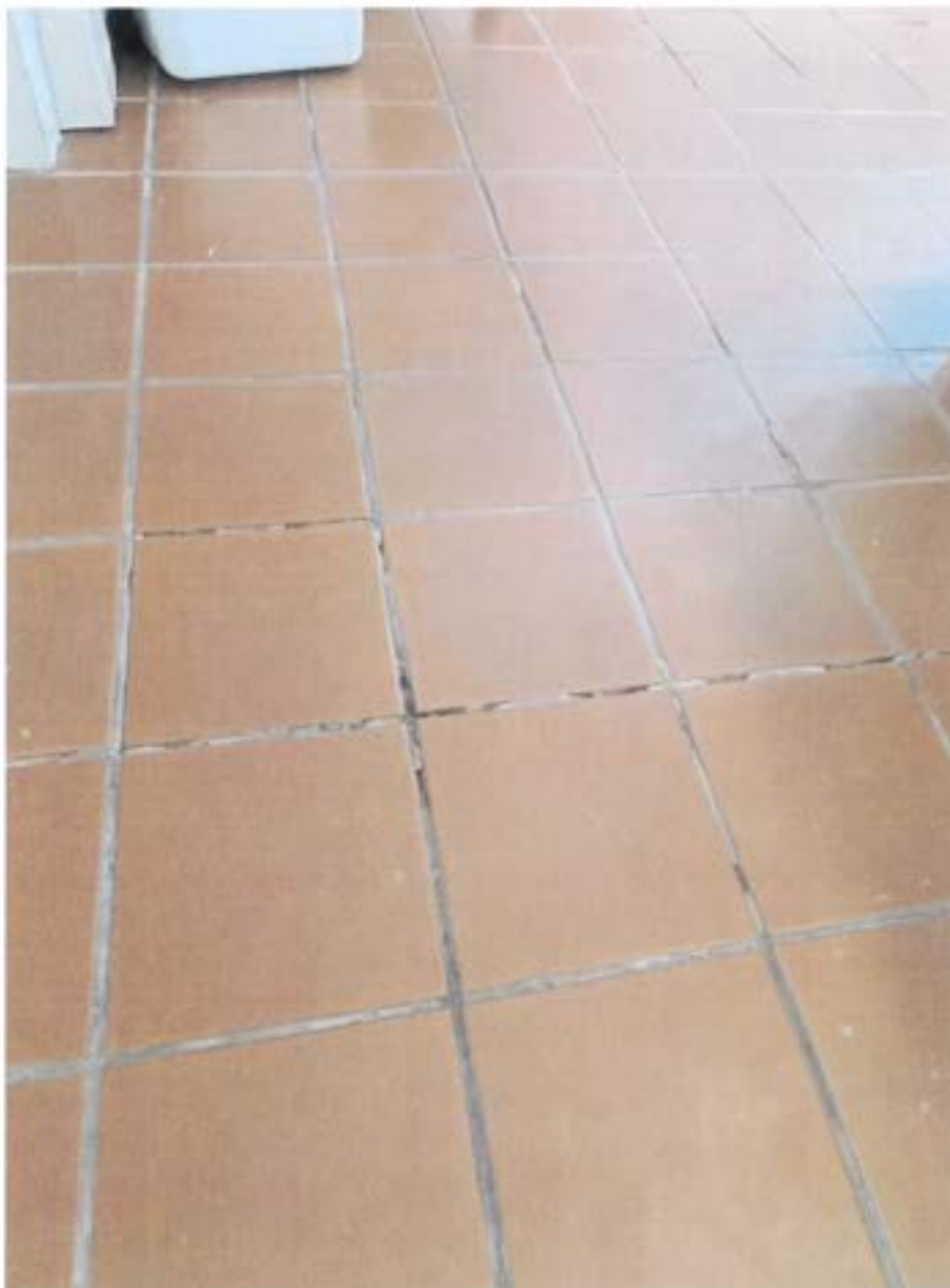
Cracked/lifting tile
