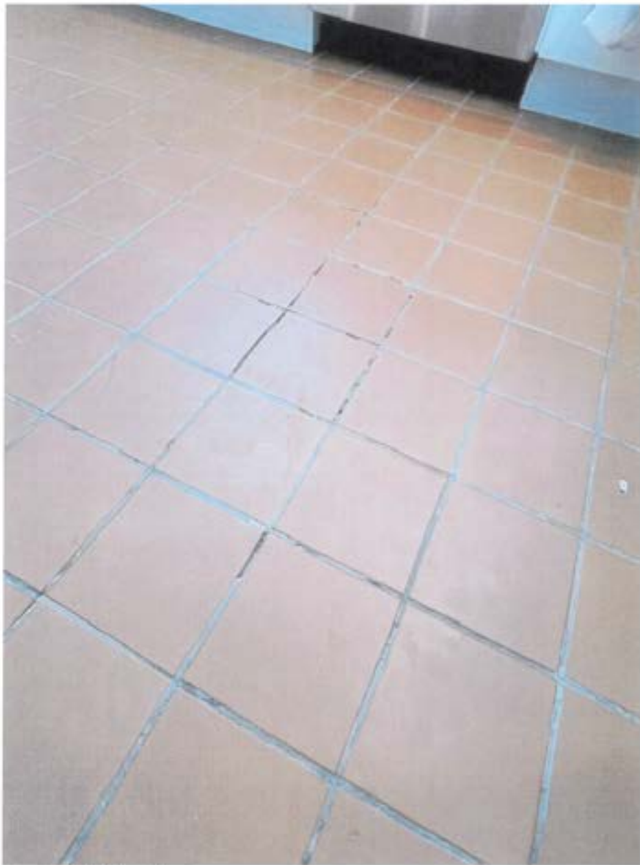
Cracked/lifting tile
