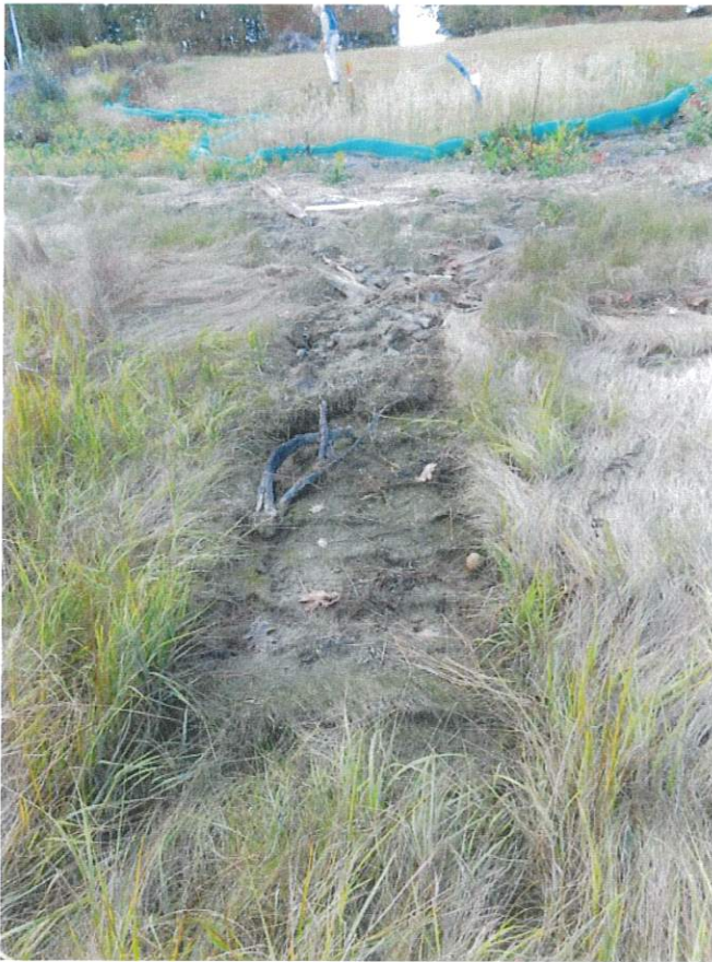
57 TON EXCAVATOR DRIVEN ON THE SALT MARSH WITHOUT TIMBERMATS. CATEPILLAR TRACKS MARK DEAD AREAS OF SALT MARSH.
