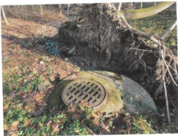
Figure B.5: Close-up of storm drain showing erosion from storm events
