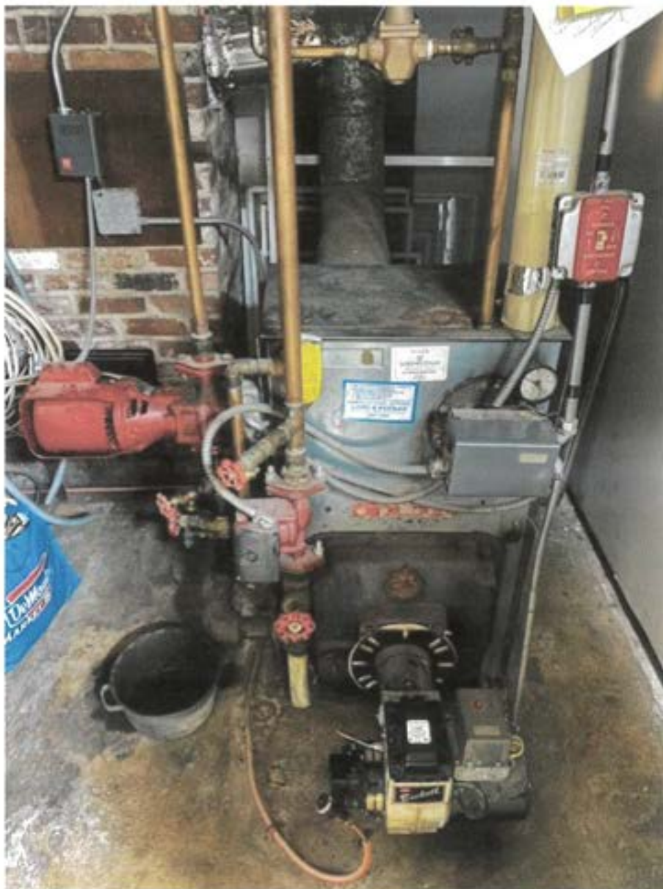
Figure D.1: Boiler (approximately 40+ years old and in need of replacement)
