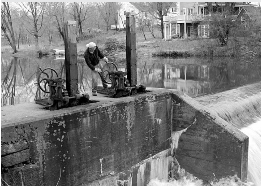
Town Engineer David Cedarholm begins the process of draining the Mill Pond in preparation for and investigation of the dam's concrete issues. ANDREA BODO PHOTO
