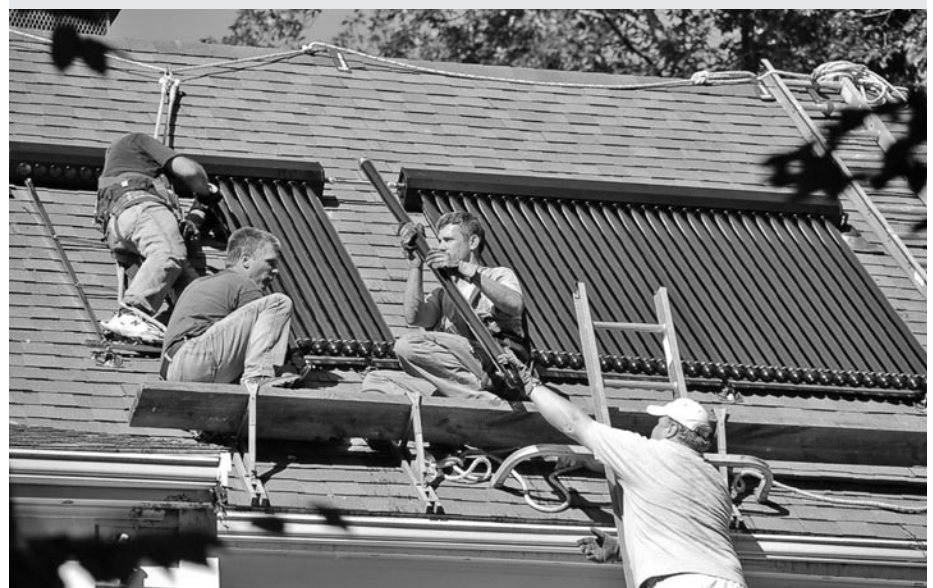
Local citizens install a solar hot water heater on a house in Durham. KEVIN GARDNER PHOTO
