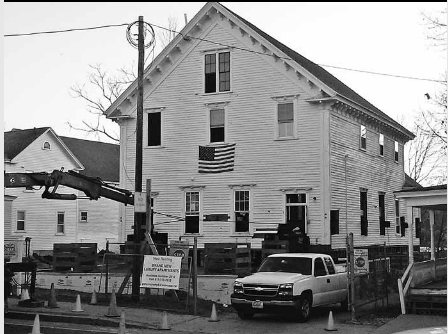
In early November, the historic Grange structure was moved forward to a new foundation adjacent to the sidewalk on Main Street. Photo Courtesy of Todd I. Selig
