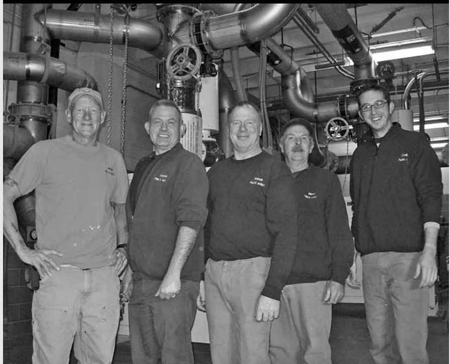
Wastewater Division (l-r): Daniel (Max) Driscoll, Daniel Peterson, Superintendent; Steve Goodwin, Lloyd Gifford and Nicholas Shonka. Photo Courtesy of Department of Public Works
