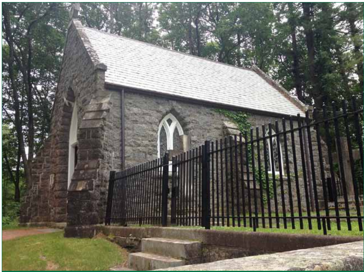
In 2013, much needed renovations were completed on the Smith Chapel (above), a favorite site in Durham for wedding ceremonies to be held. The scope of work on the chapel included a new slate roof and copper gutter, down spouts and ridge cap, stain glass window rehabilitation, brick walkway rehabilitation, new electric service/lighting, custom design trim work repair, landscaping, exterior painting, and cleaning/polishing of all brass items. COURTESY ANDREA BODO
