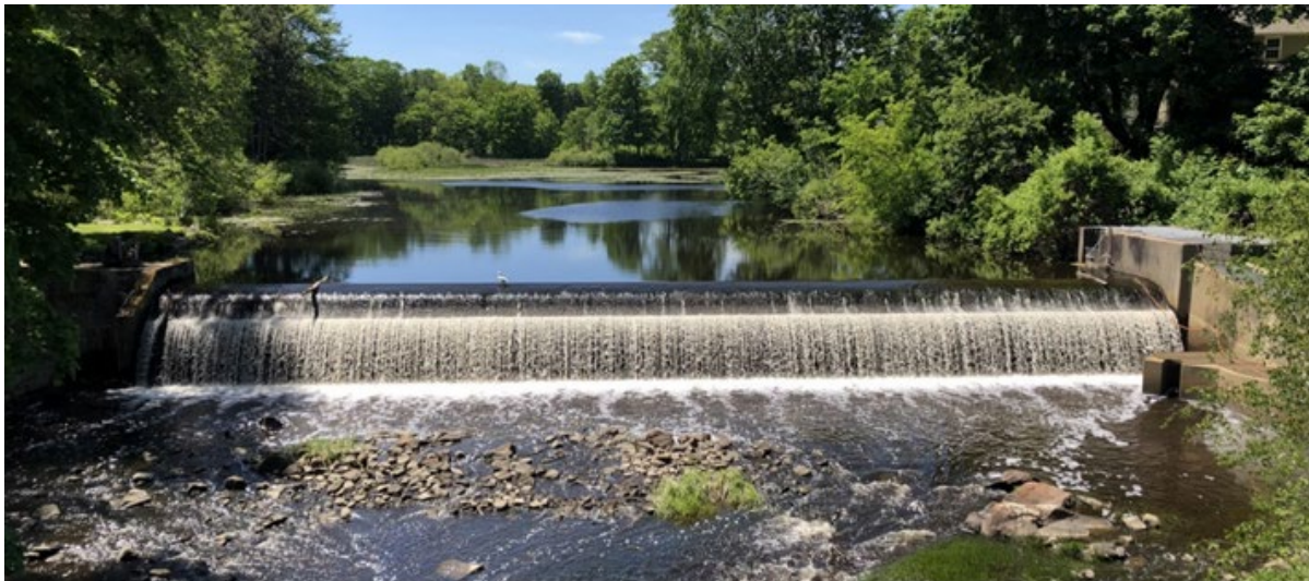
Mill Pond Dam – Photo Credit: VHB
