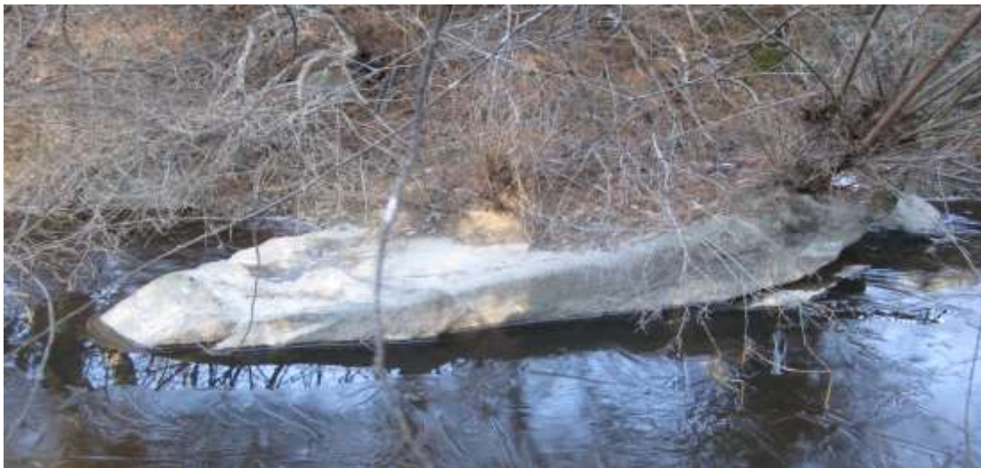
Image 29: Remains of stone bridge abutment over Dirty Brook, now LaRoche Brook, east of the tracks
