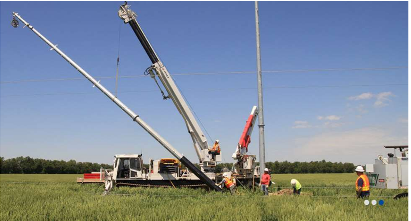
Crane on tracks maneuvering assembled pylon
