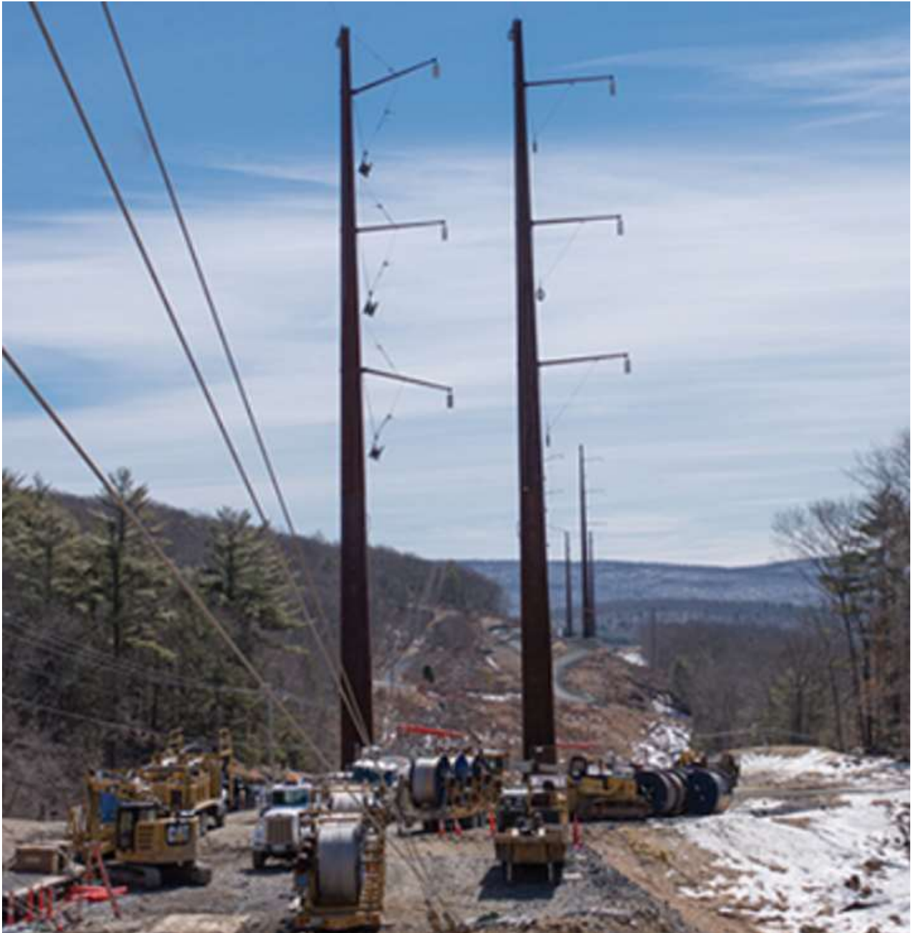
Transmission lines construction, Eversource website
