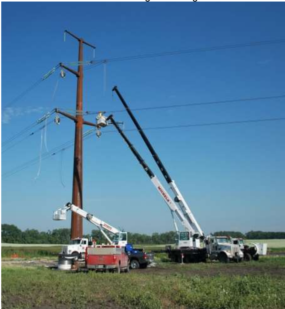
Multiple cranes at job site
