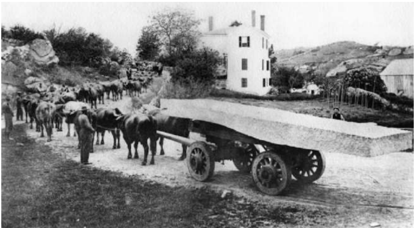
Image 16: Fifteen yoke of oxen hauling a 12 ton slab of granite from the Cape Ann Quarry in 1870
