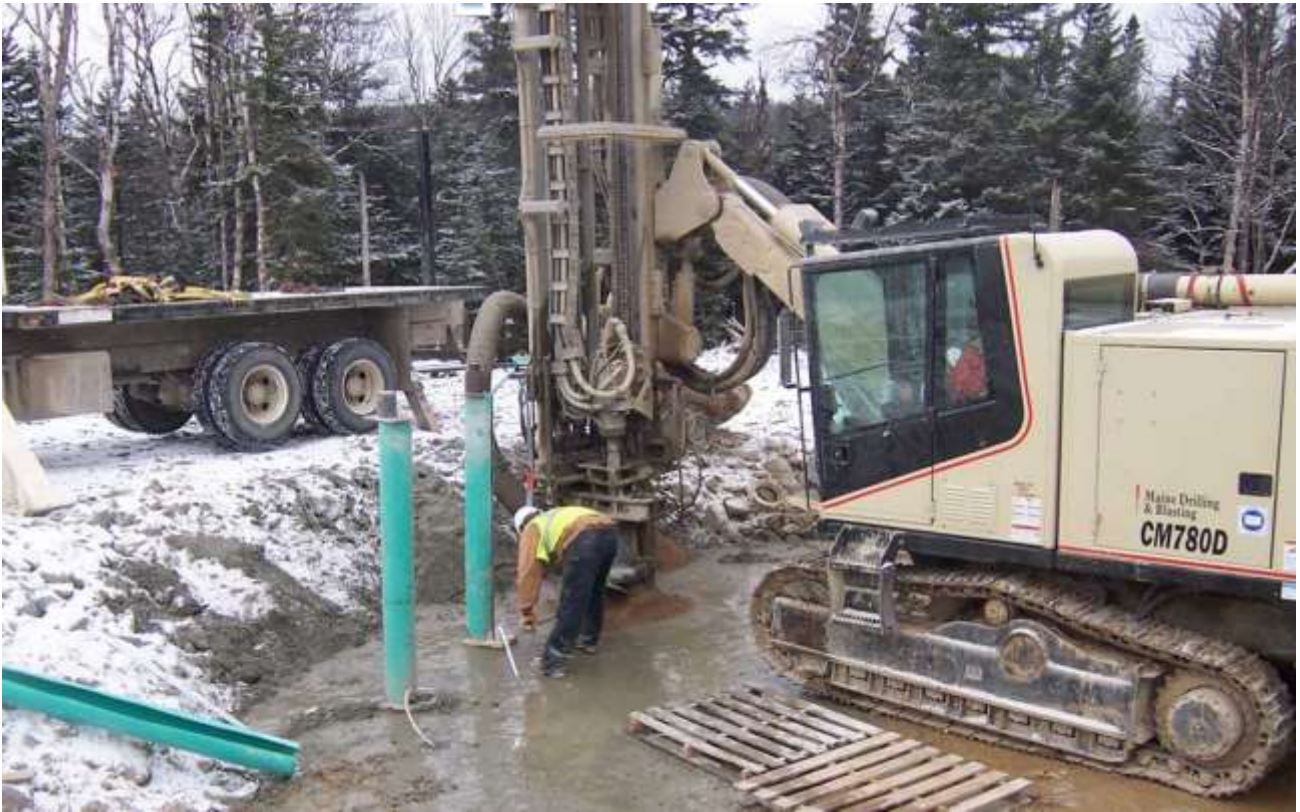
Maine Drilling & Blasting
