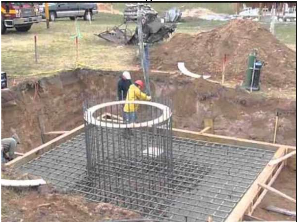
Reinforced pole base
