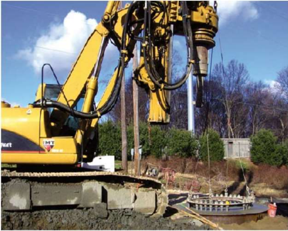
Assembling pole base
