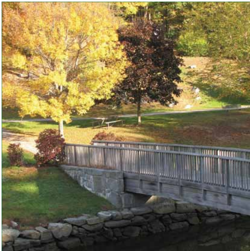
Footbridge over the Oyster River. Courtesy Noelle Khleif
