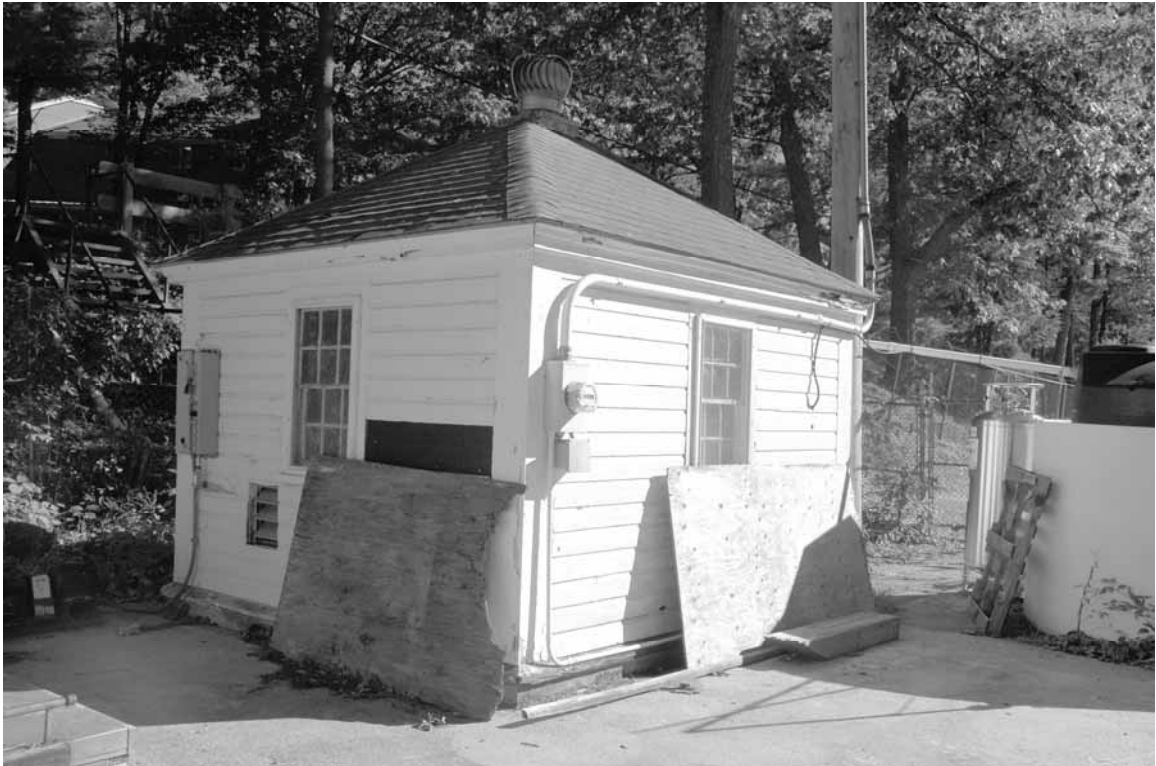
Photo 28: Rear of filter house
