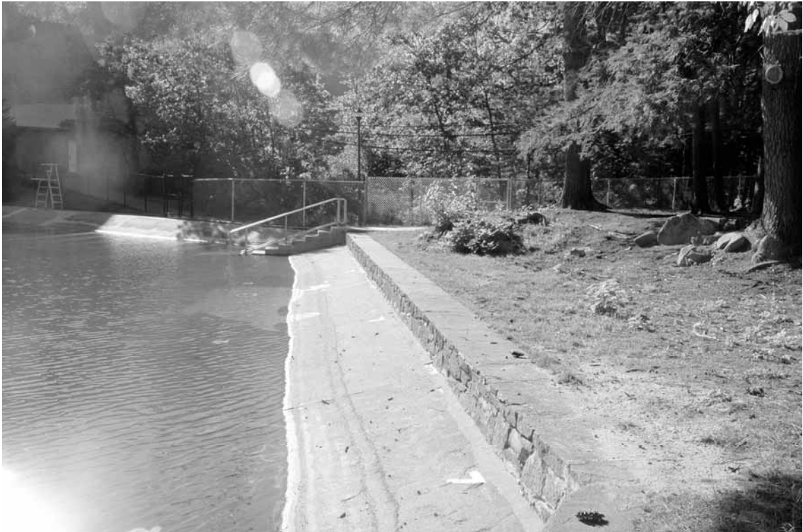
Photo 19: Northern edge of pool, rebuilt stone wall and concrete slope
