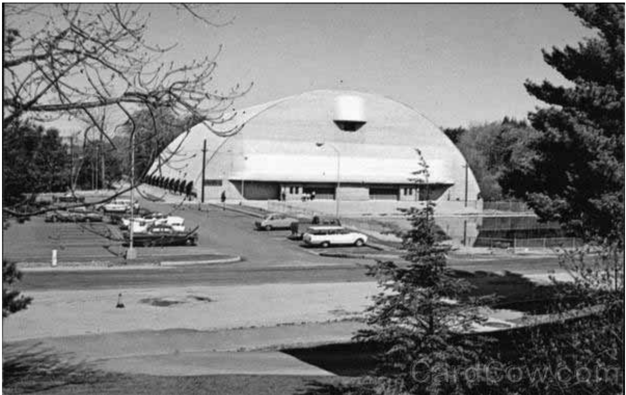
1970s postcard view of Snively Arena from across Edgewood Road, facing north ( http://www.cardcow.com/391659/university-new-hampshire-snively-arena-outdoor-swimming-pool-durham )
