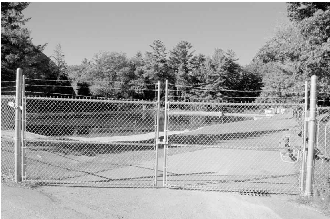
Photo 37: Service entrance gate from parking lot
