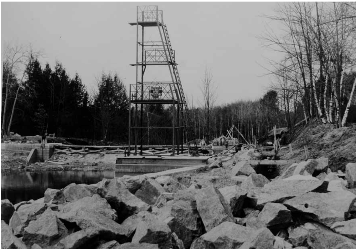
April 1937 - Quarried stone piled near dive tower, dam at rear (UNH Archives 12712a)
