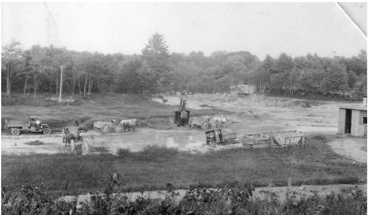
1924 Pond construction, looking toward dam (Collection Durham Historic Association)
