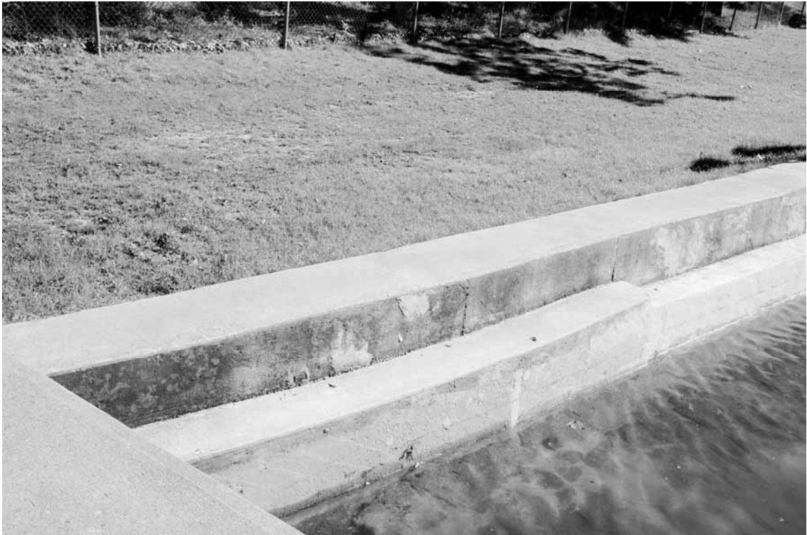
Photo 15: Pool wall at diving platform
