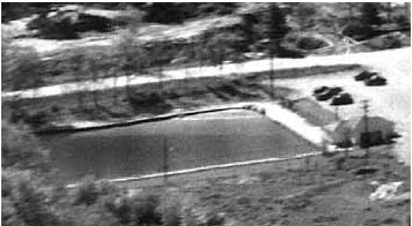
1954 detail, facing south toward Edgewood Road
