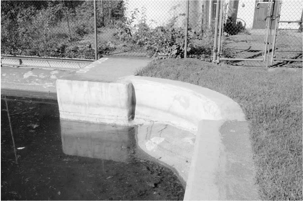
Photo 21: Northeast corner of pool, at Dam
