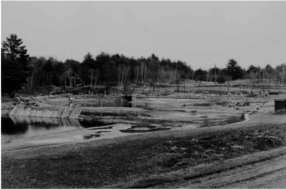
April 1937 beginning construction of dike, looking east toward pool area, Edgewood Road in back (UNH Archives 12712b)
