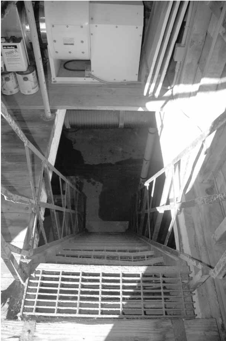
Photo 31: Stairs to lower level
