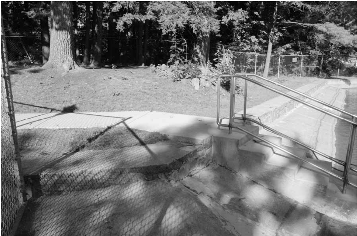
Photo 18: North edge of pool, new access point
