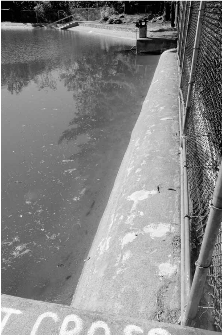
Photo 23: Top of dam
