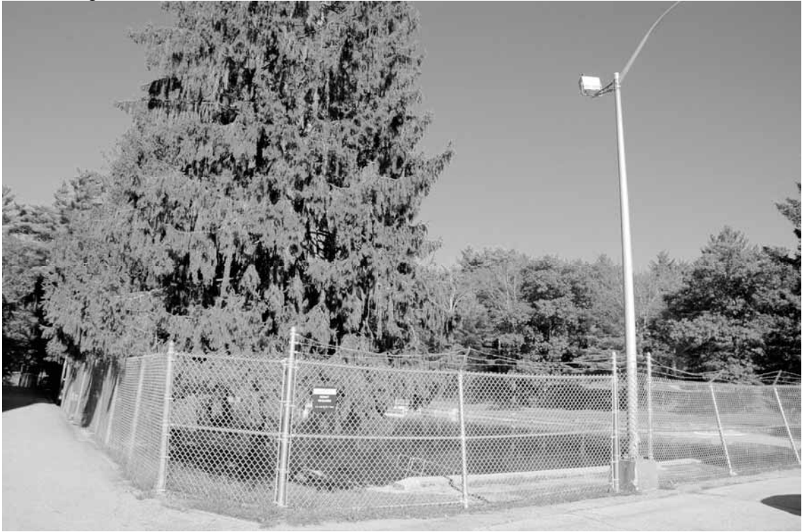
Photo 34: Pool perimeter fence from parking lot
