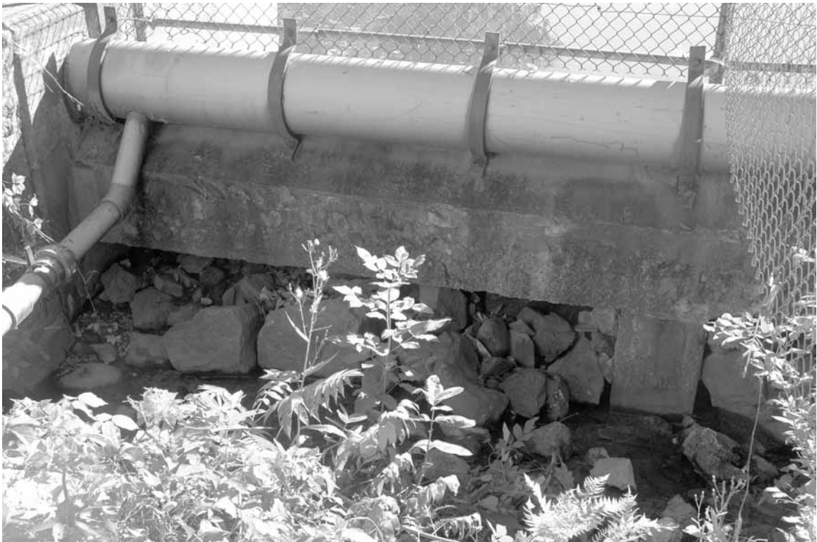
Photo 25: Back side of dam
