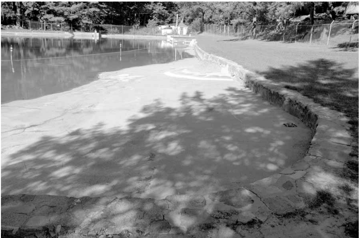
Photo 6: Southeast edge of pool from Minnow beach area, now concrete, looking toward diving platform and treatment plant
