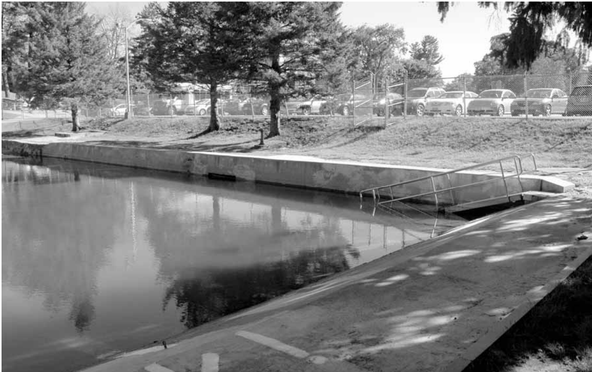
Photo 10: Newly cemented southwest wall
