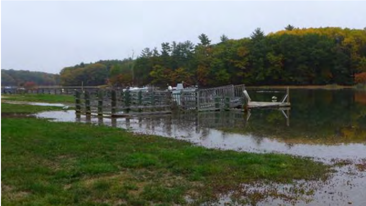
King Tide Flooding at Old Town Landing – Photo Credit: SRPC
