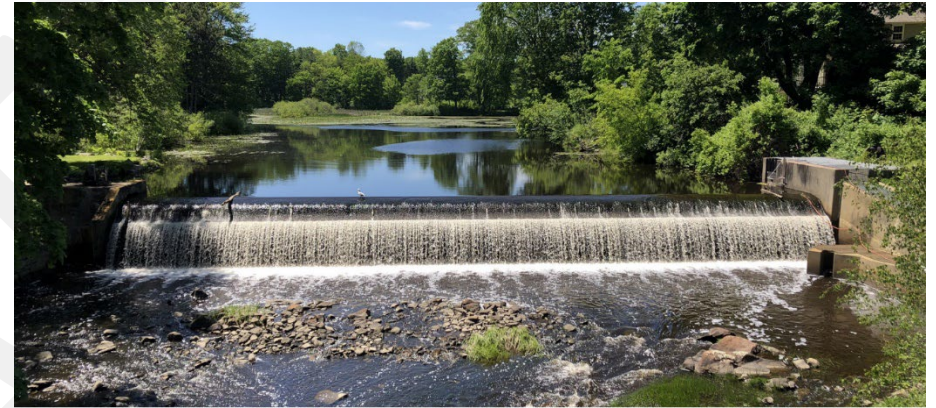
Oyster Ricer Dam at Mill Pond (Photo Credit: VHB)
