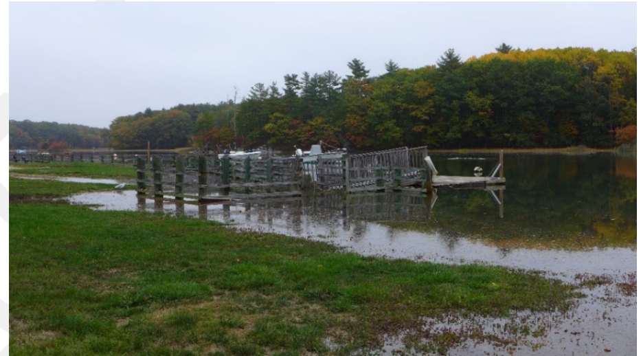
Coastal Flooding at Town Landing during 2017 King Tide Event (Photo Credit: Strafford Regional Planning Commission)
