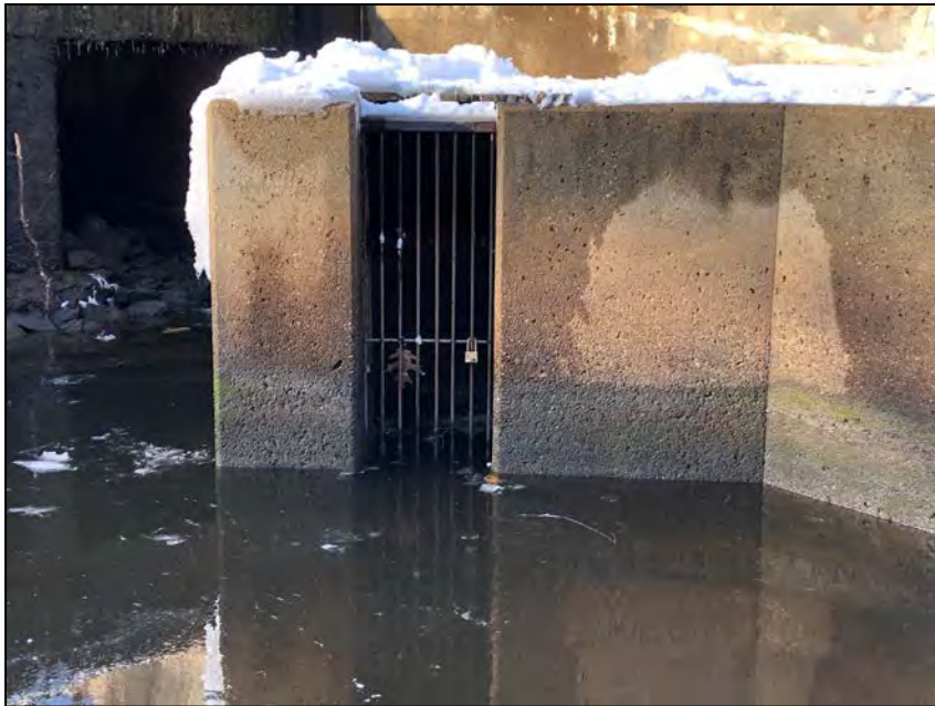
Photo No. 57: Outlet of the fish ladder.
