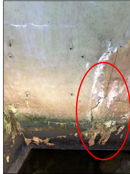
Photo No. 10: Right side of the upstream sloped ceiling. Note the delamination of the repairs.
