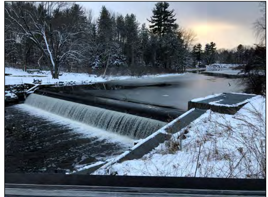
Photo No. 60: Mill Pond Dam and the impoundment from the top of the bridge at Newmarket Road.
