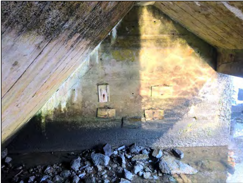
Photo No. 37: Left wall. Note repairs covered with timber falsework.
