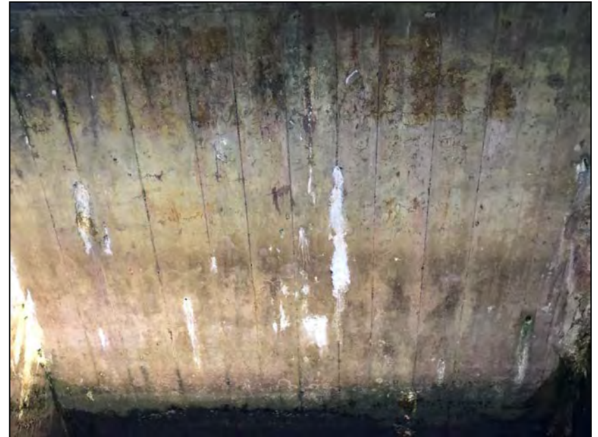
Photo No. 20: Overview of the upstream sloped ceiling.
