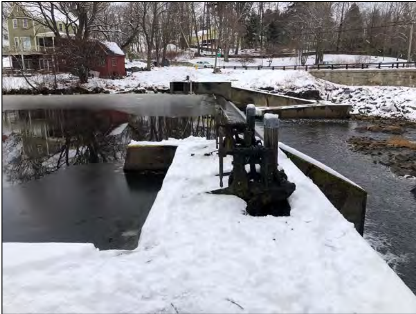
Photo No. 45: Overview of the top of the low-level outlet structure.
