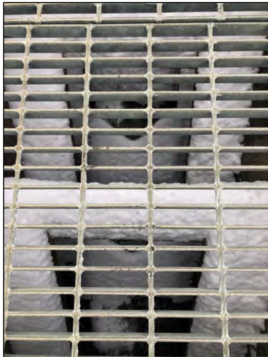
Photo No. 55: Inside of the fish ladder.
