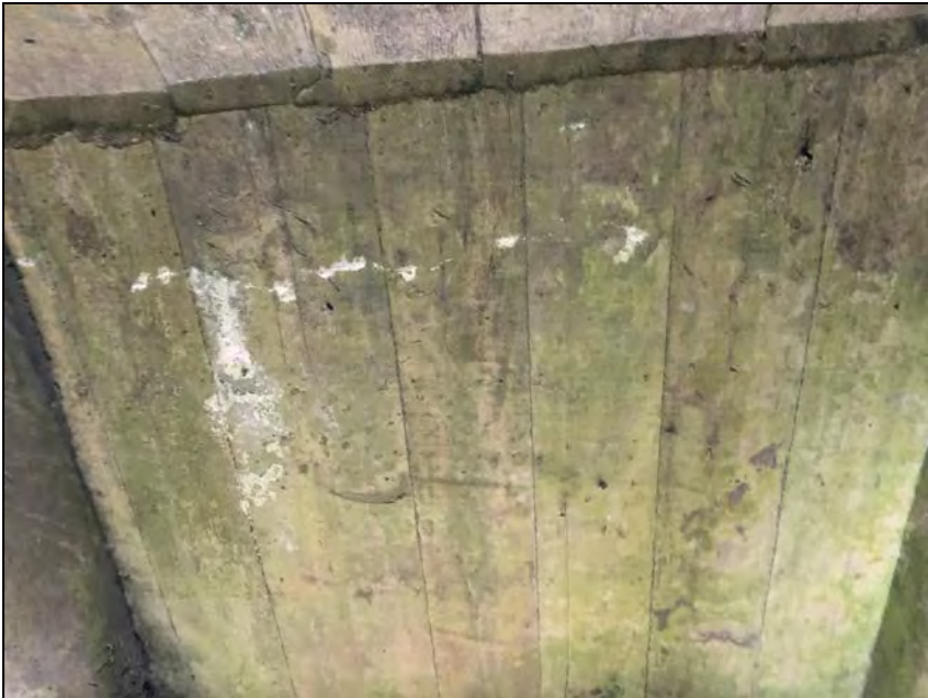
Photo No. 43: Downstream sloped ceiling.
