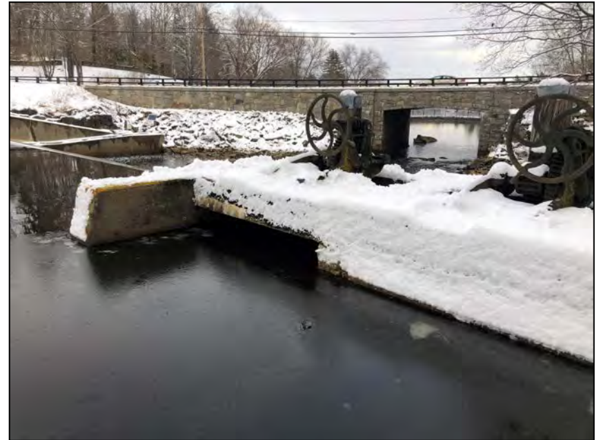
Photo No. 46: Intake of the gate structure.
