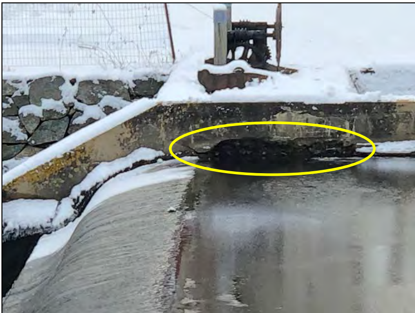
Photo No. 3: Scour on the left side of the right training wall upstream of the spillway crest.
