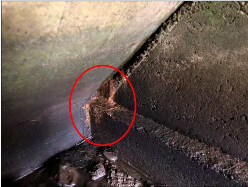
Photo No. 41: Upstream left corner of the cell with iron oxide staining.
