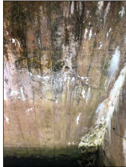
Photo No. 30: Delamination and staining along the joint between the ceiling and the left wall.
