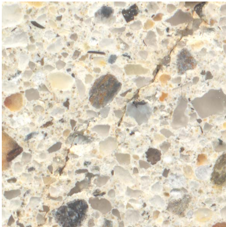
Figure 2 Section A close up of Figure 1 core #1
