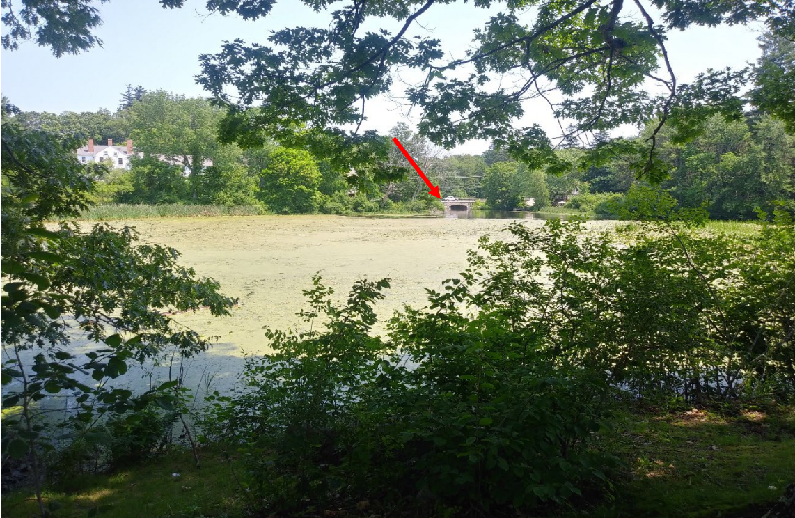
Photo 9: View east of Mill Pond taken from Mill Pond Park. Note the Newmarket Road bridge in the background (red arrow). 07/12/2023.
