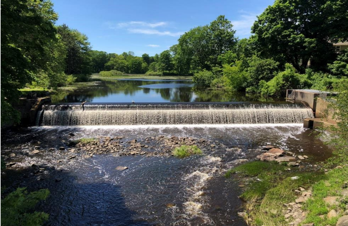
Photo 1: View west of the Oyster River Dam taken from Newmarket Road. Date uncertain.
