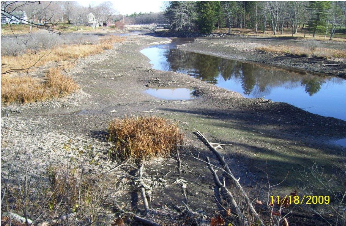
Photo 12: View east of the Oyster River within the drained Mill Pond impoundment during a drawdown. 11/18/2009.
