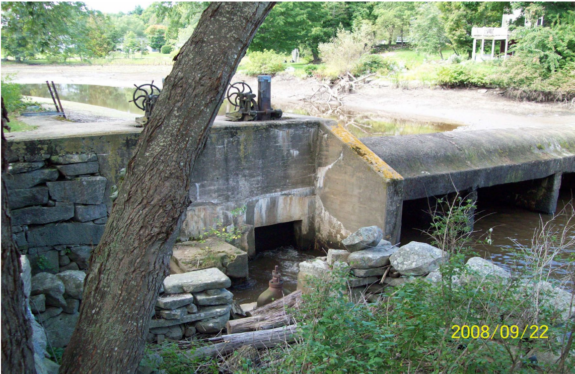
Photo 6: Closeup view west of the mill remnants and southern dam abutment. 09/22/2008.
