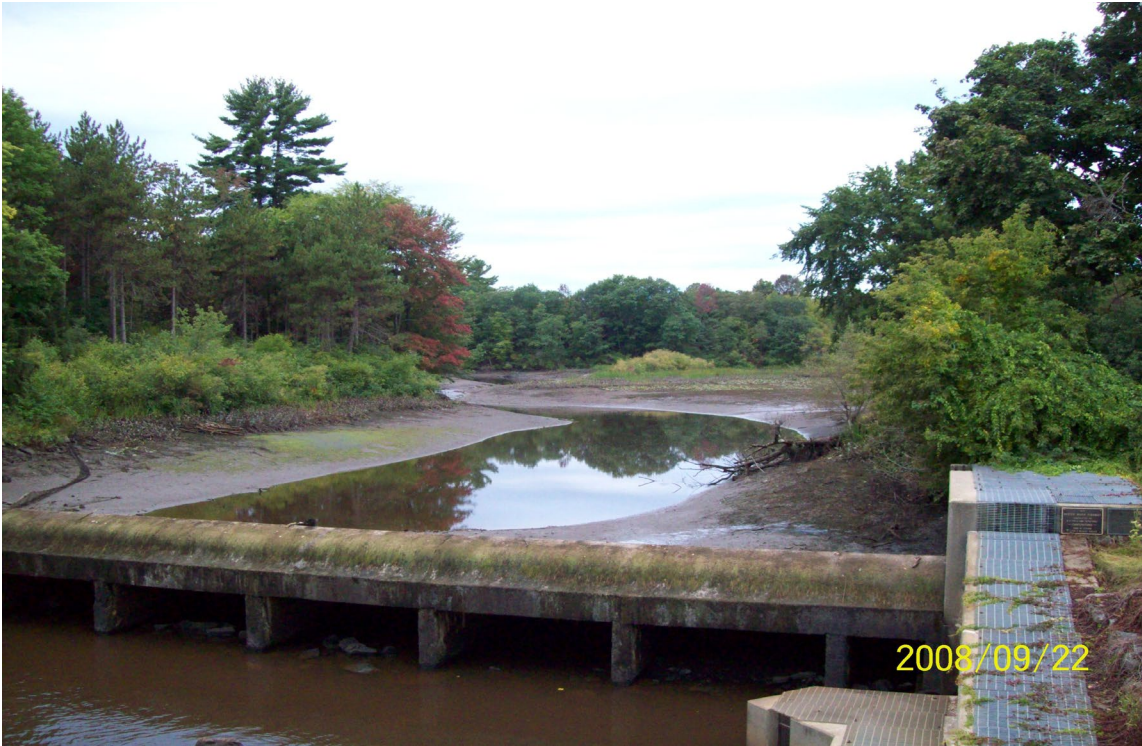
Photo 5: View west of the dam and surrounding area during a drawdown. 09/22/2008.
