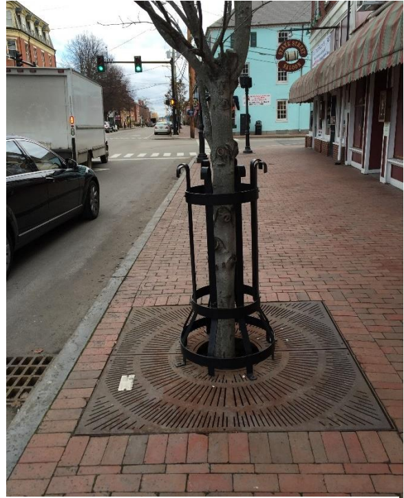
Figure 12 - Stormwater Tree Planter Combined with Catch Basin
