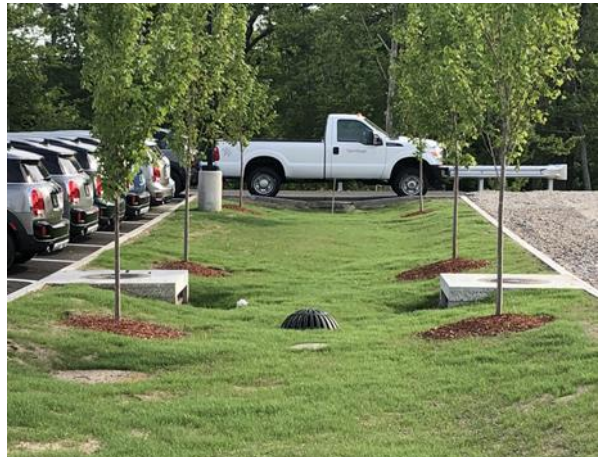
Figure 13: Parking Lot Bioretention
