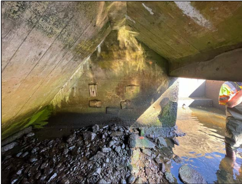
Photo No. 37.: Left Wall: Note repairs covered with timber falsework.
