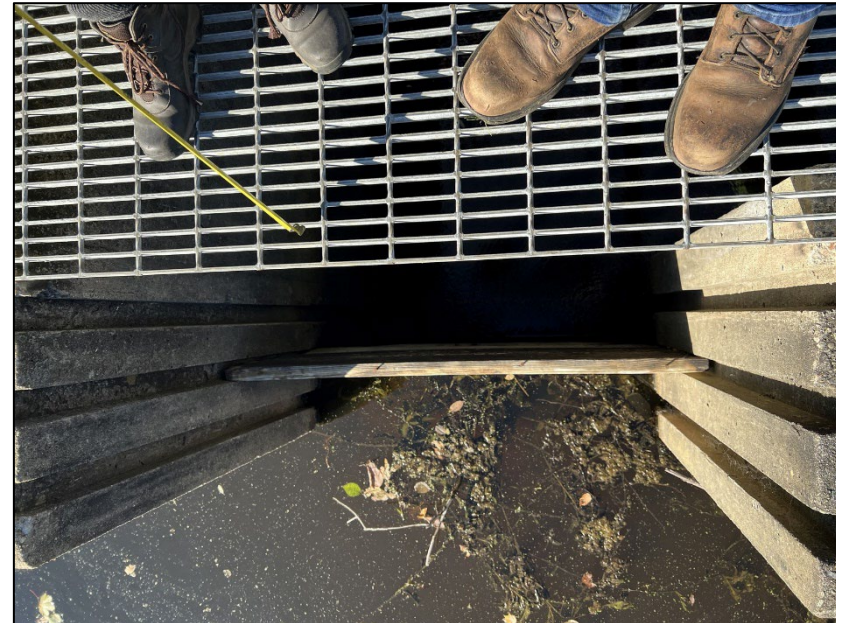
Photo No. 52.: Upstream end of the fish ladder.
