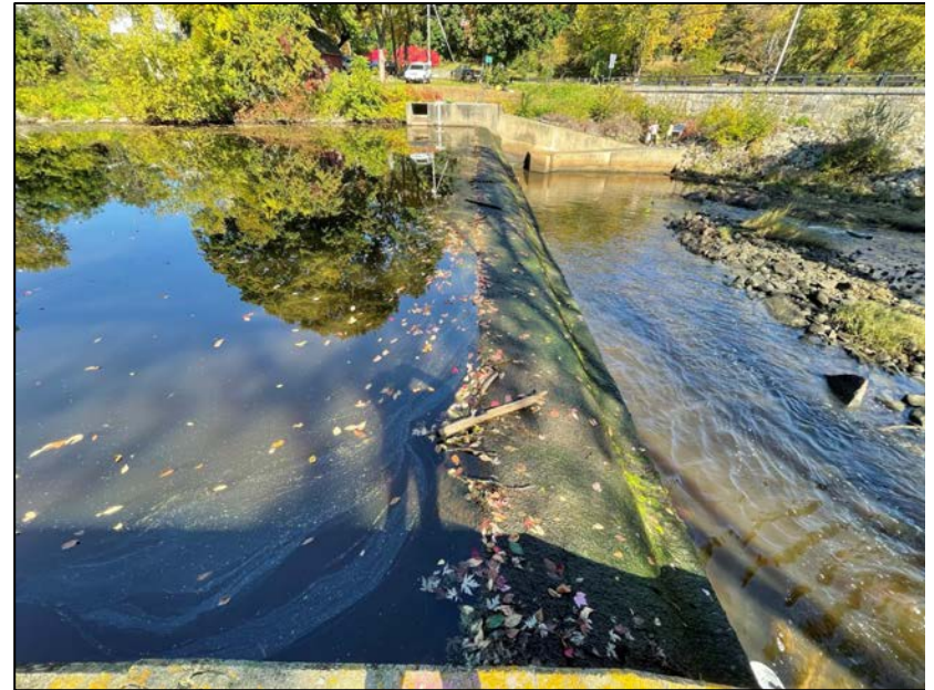
Photo No. 3.: View of the spillway crest
