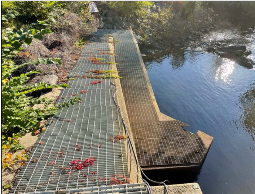
Photo No. 53.: Overview of the top face of the fish ladder.
