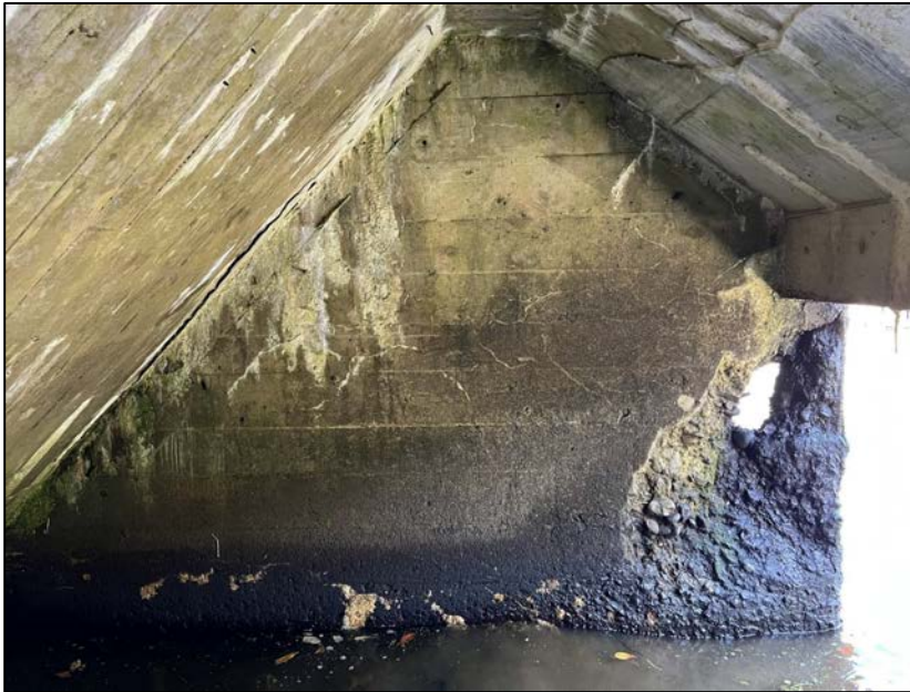
Photo No. 9.: Left interior wall
