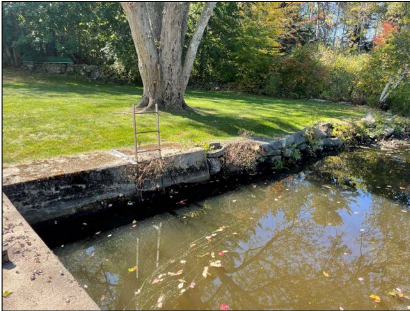
Photo No. 45.: Right abutment upstream of the low-level outlet.
