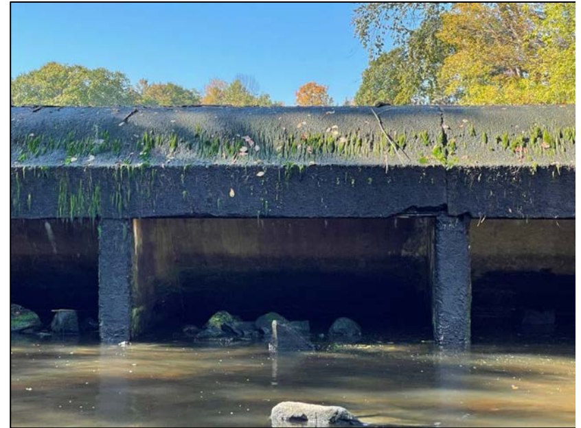
Photo No. 31.: Overview of the downstream face of the Cell.
