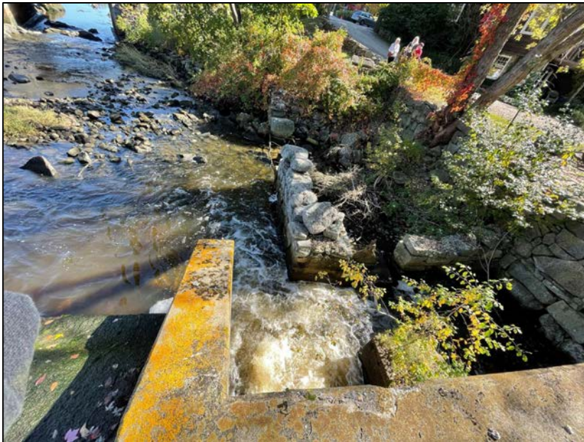
Photo No. 50.: Remnants of mill foundations downstream of the low-level outlet.
