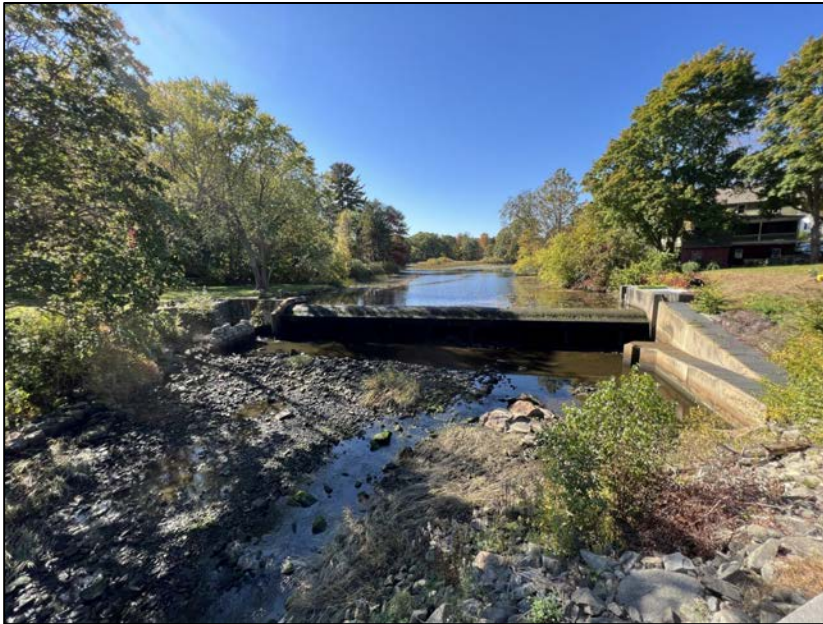
Photo No. 1.: Overview of the downstream side of the dam.
