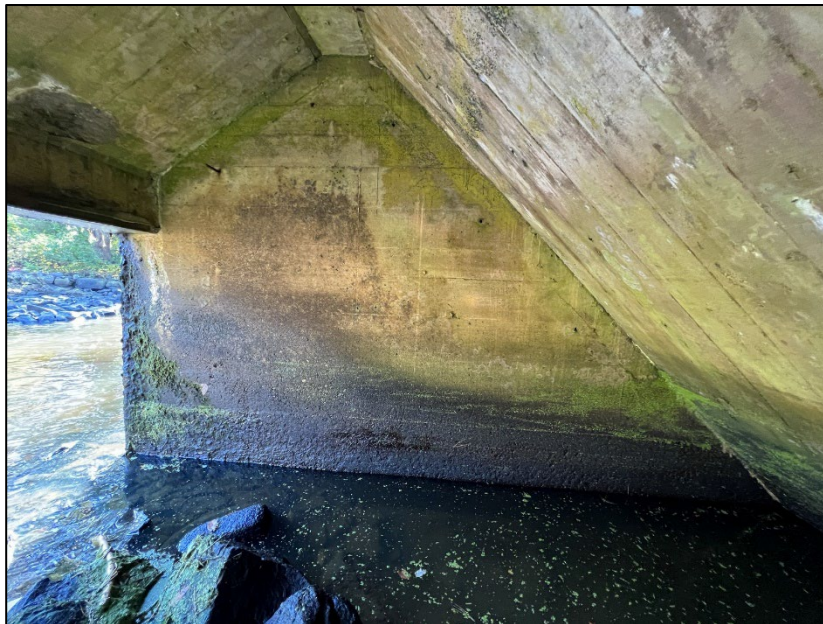
Photo No. 30.: Right Wall. Concrete in fair condition.
