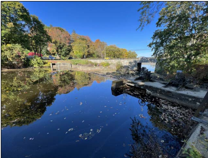
Photo No. 2.: Overview of the upstream side of the dam.
