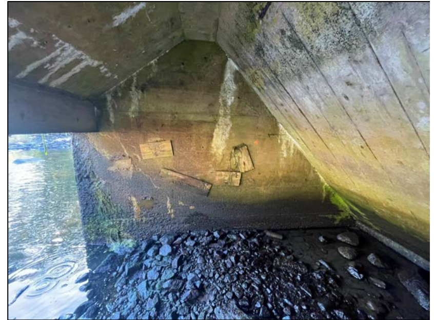
Photo No. 39.: Right wall
