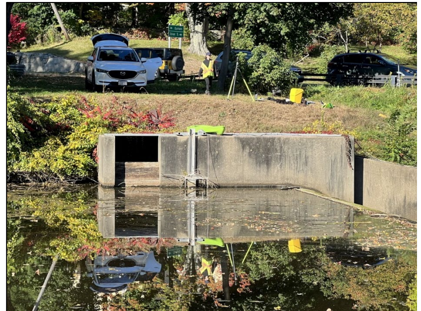
Photo No. 4.: View of the left abutment
