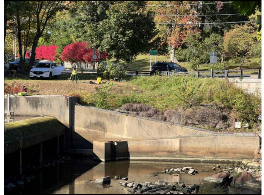
Photo No. 51.: Overview of the fish ladder at the left abutment.
