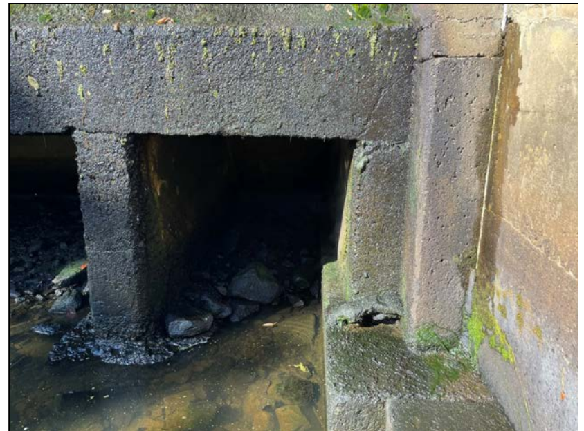
Photo No. 44.: Downstream face of Cell 9.
