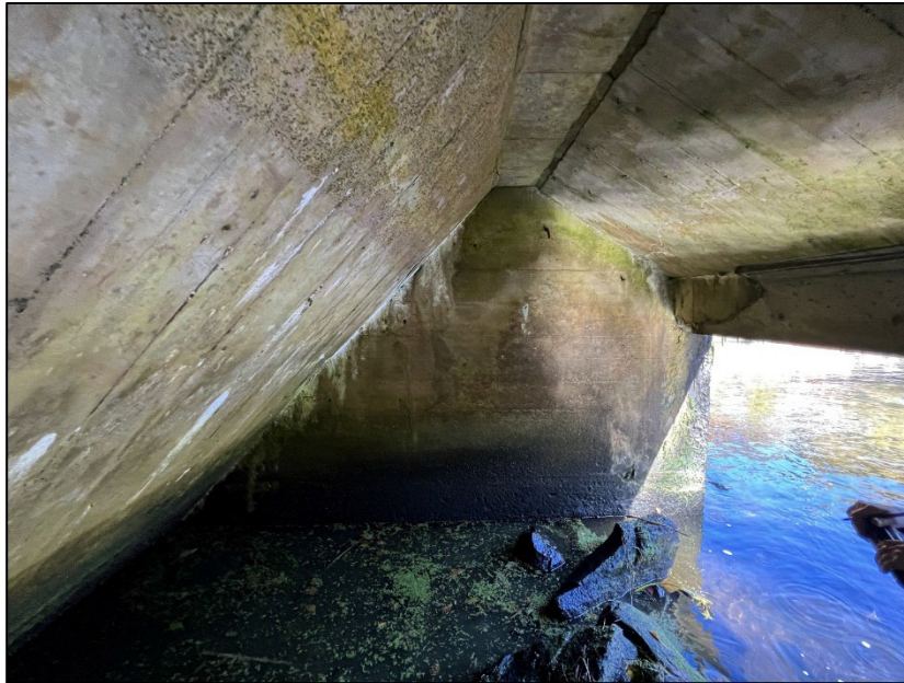
Photo No. 25.: Left Wall. Note scour and light spalling along the downstream end of the wall and approximately 1-foot above the waterline at the time the photo was taken.
