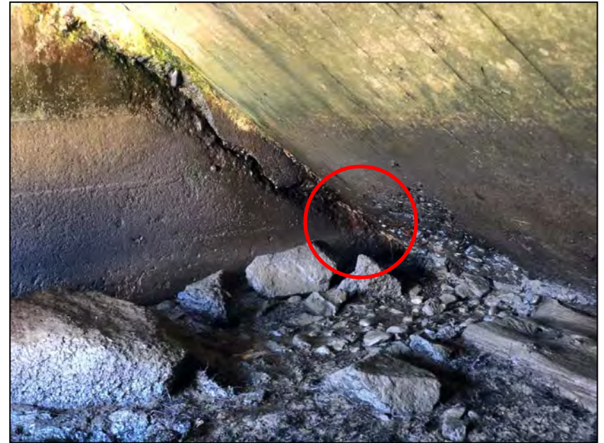
Photo No. 22: Large crack and spall along the right wall with iron oxide staining on the upstream end.
