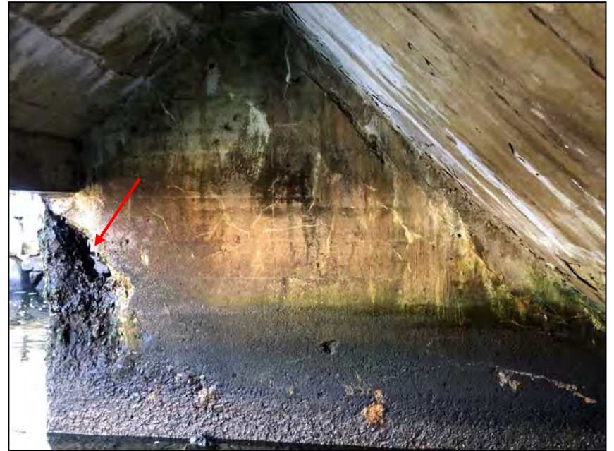
Photo No. 14: Right Wall. Note the section loss on the downstream end.
