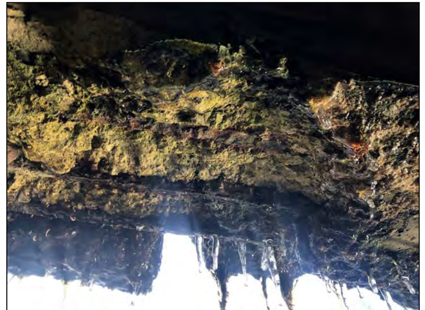
Photo No. 32: Spalling with debonded rebar on the underside of the downstream most ceiling (ceiling face no. 1).
