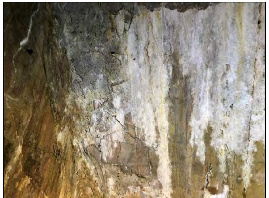
Photo No. 16: Delamination on the upper part of the upstream sloped ceiling (ceiling face no. 5).
