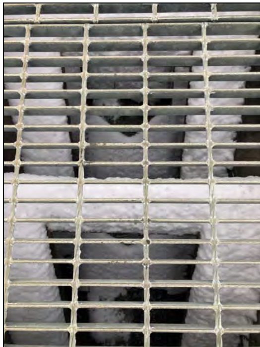
Photo No. 55: Inside of the fish ladder.
