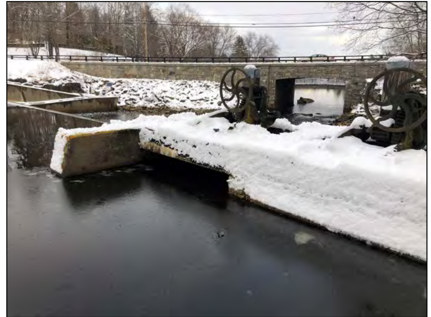
Photo No. 46: Intake of the gate structure.
