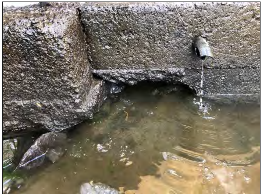
Photo No. 56: Scour and undermining underneath the right training wall of the fish ladder. Note void probed up to 3 feet.
