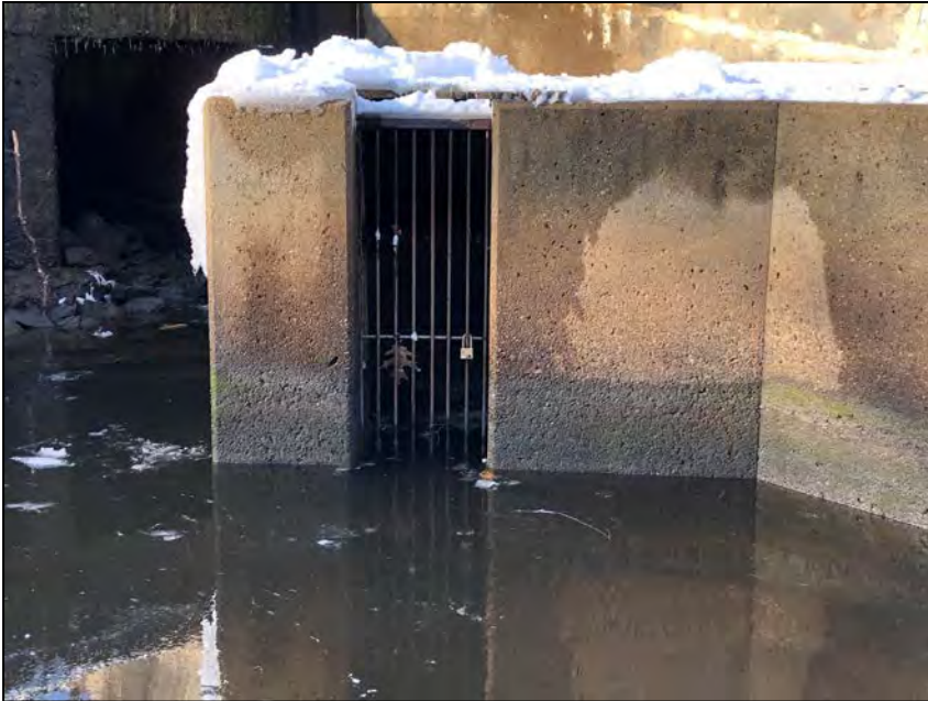
Photo No. 57: Outlet of the fish ladder.
