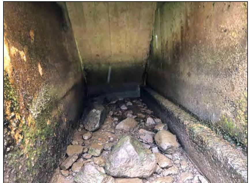
Photo No. 44: Overview of the cell.
