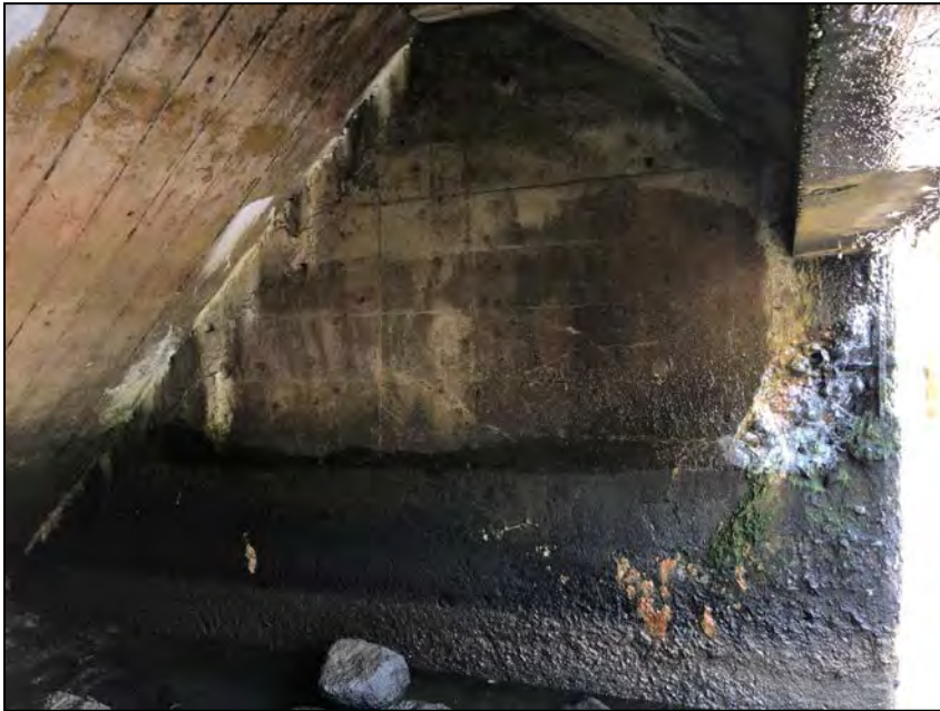
Photo No. 21: Left wall. Note debonded rebar and spalling on the downstream end.
