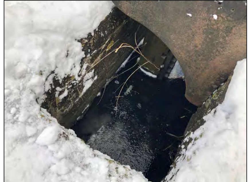
Photo No. 48: Inside of the top of the gate opening. Note irregular concrete typical in both gate openings.
