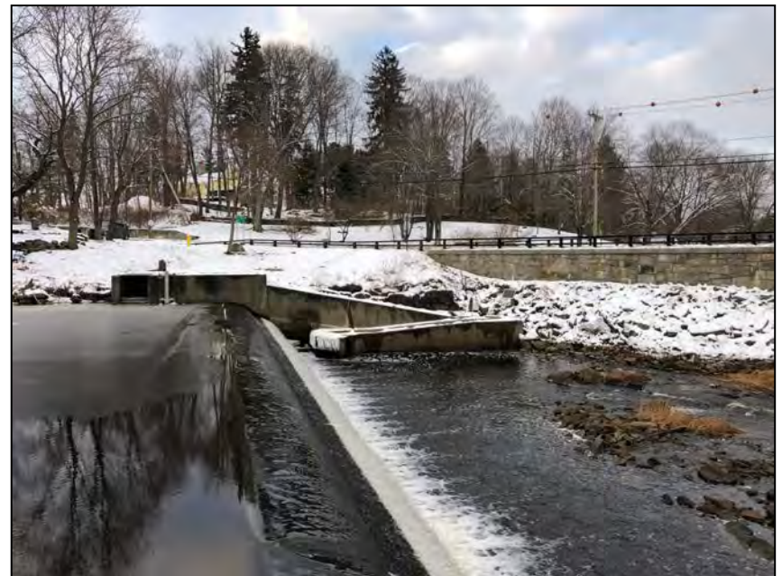
Photo No. 4: View of the left end of the primary spillway and training wall.
