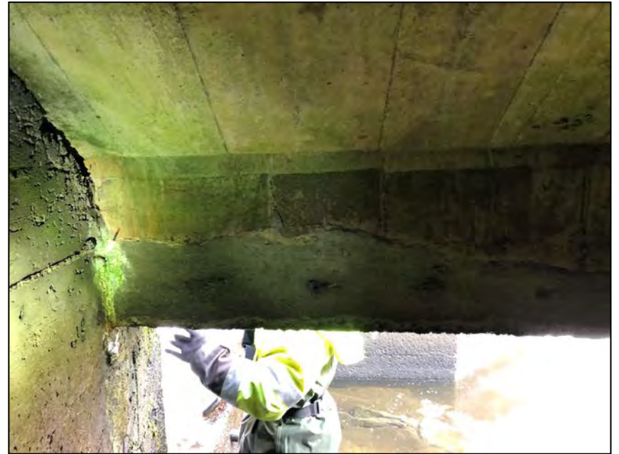
Photo No. 42: Repair on the downstream side of the cell (ceiling face no.2).
