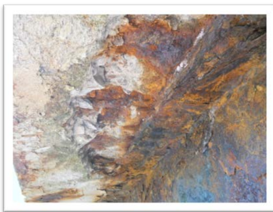
Underside of Downstream Curb
