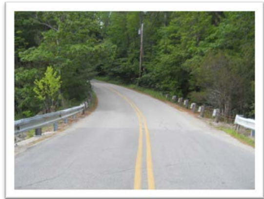
Damaged Approach Rail
