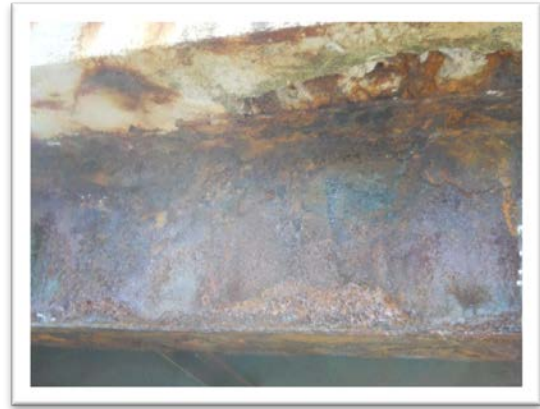
Downstream Exterior Girder
