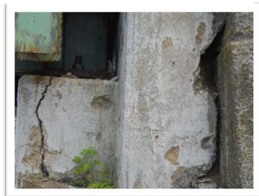
North Corner of West Abutment
