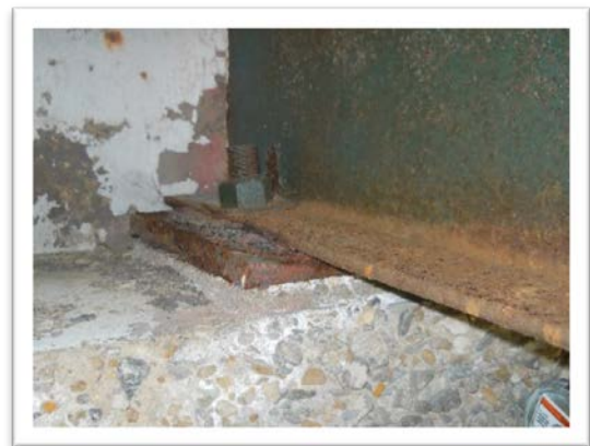
Typical West Bearing Plate
