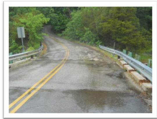
Drainage on Bridge Looking East
