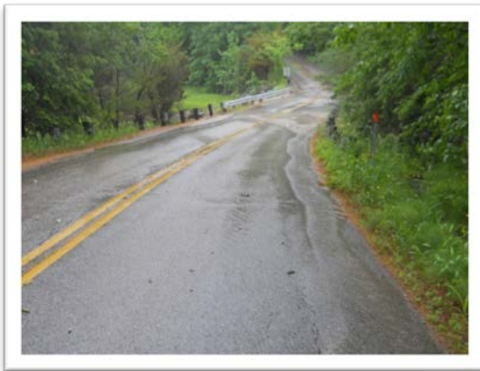
Drainage Flow Looking East
