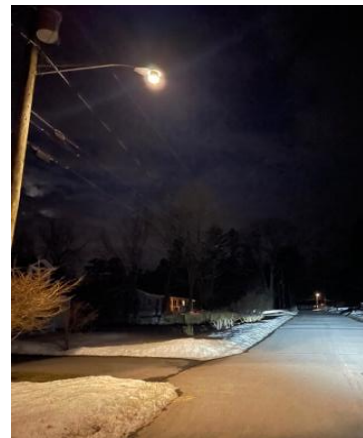
Figure 1: A streetlight in a residential area which is shielded to reduce light trespass into residential properties.
