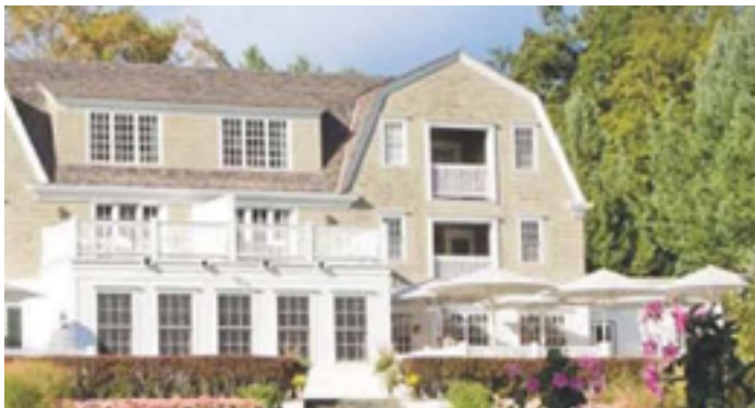
Example of small frontage building to screen mass and significant breaks in overall volume.
