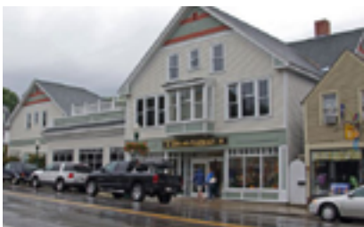
Larger gables flank this roof deck to provide elevated outdoor space.
