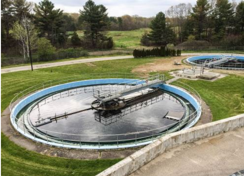
Clarifying tank at wastewater center (Photo Credit: Town of Durham)
