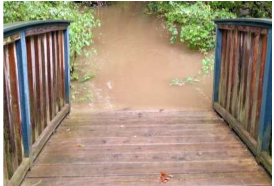
Access to the College Brook Footbridge blocked by flood waters
