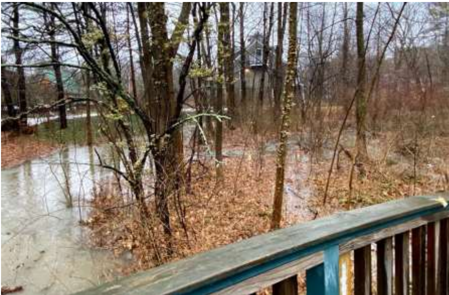
The College Brook Footbridge overlooking typical brook flooding
