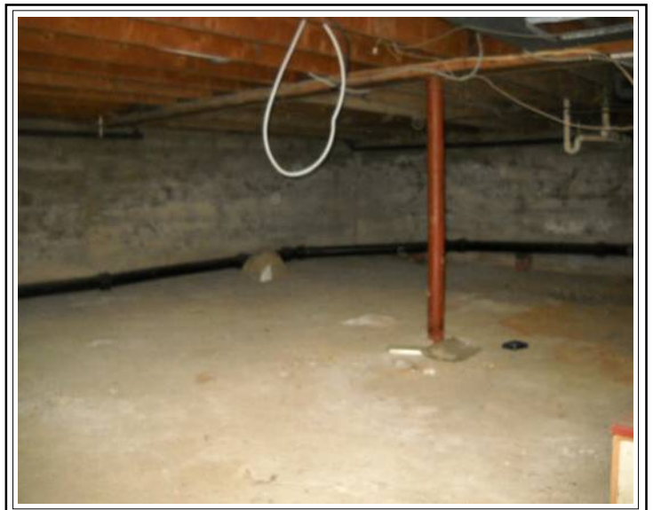
Basement showing crawl space
