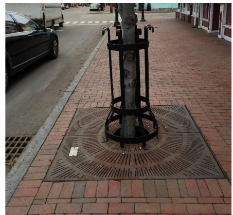
Figure 12 - Stormwater Tree Planter Combined with Catch Basin
