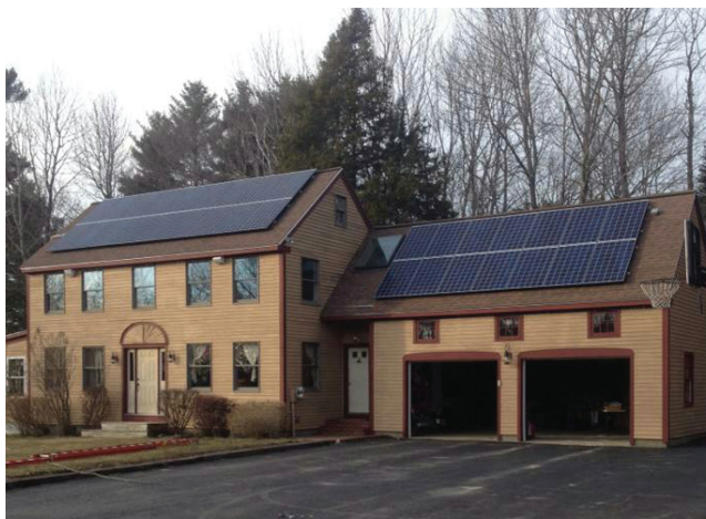
A solar photovoltaic installation, such as this one for a customer in Maine, will raise the value of the home roughly $20,000 (based on a 4-5 kW solar electric system)
