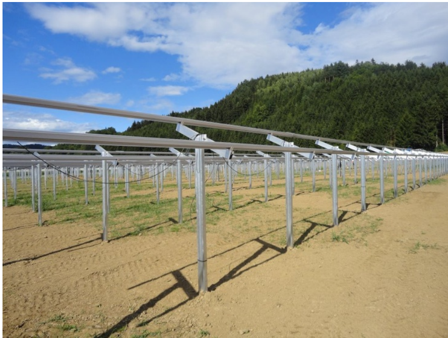
Racking equipment – prior to panel installation.
