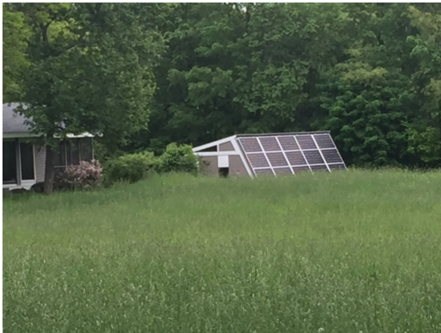
Residential Ground mounted system.
