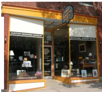
The storefront in Dover is open and clear and the recessed entry draws in customers (although it would be preferable to break up the size of the glass with a few mullions). (135)
