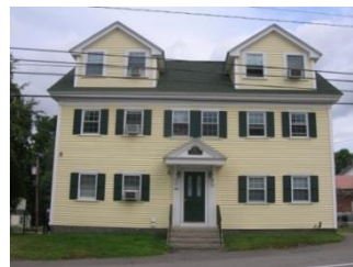
The dormers are out of proportion relative to the rest of the house resulting in an ungainly, top-heavy appearance. (58)
