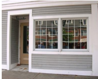
The windows are squat/square and the fake grille impedes visibility. Clapboards are generally too rustic in character to use on a storefront. (137)
