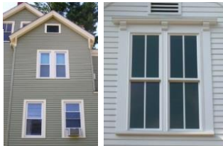
These double windows on Durham buildings are properly separated by strong, wide mullions. (85)
