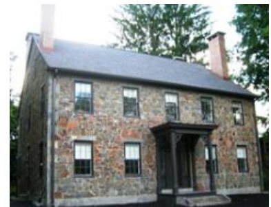
This iconic house on Newmarket Road is a rare example built with shale. (115)
