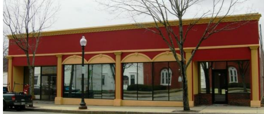
Rochester – new façade (59)
