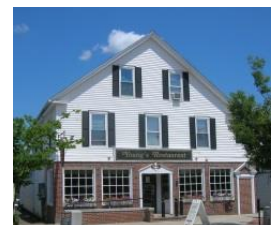
Young's Restaurant – a 2-1/2 story building (150)
