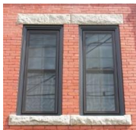
All windows in masonry buildings shall have a distinct lintel over the windows, providing structural, or at least convincing visual, support to the window opening. (86)
