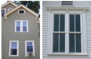
These double windows on Durham buildings are properly separated by strong, wide mullions. (85)
