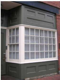
If a grille is to be used it shall be composed of real through-muntins and separate panes of glass. (133)
