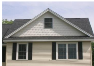
Cross gables shall rise straight from the wall below, with no extension of the roof across the bottom of the triangle. (78)
