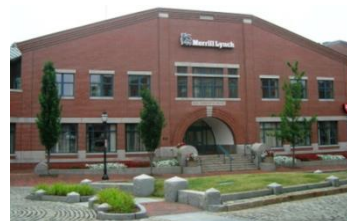
Cross gables shall rise straight from the wall below, with no extension of the roof across the bottom of the triangle. (78)
