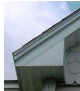
Porkchop eaves are clunky and inappropriate. (77)
