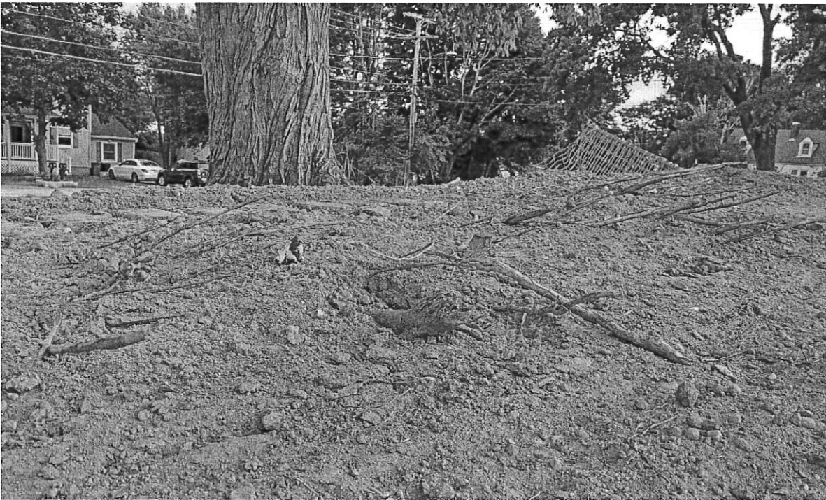
Tree B showing roots exposed by grading, some within 15 feet of trunk
