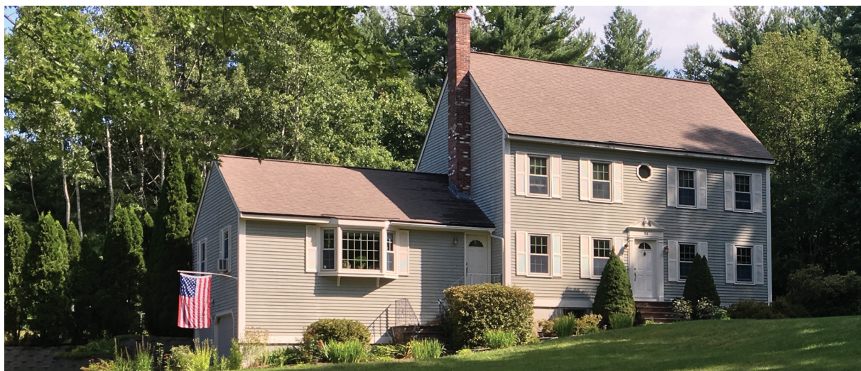
An ADU is seen attached to the left side of this home in Hollis, NH.
