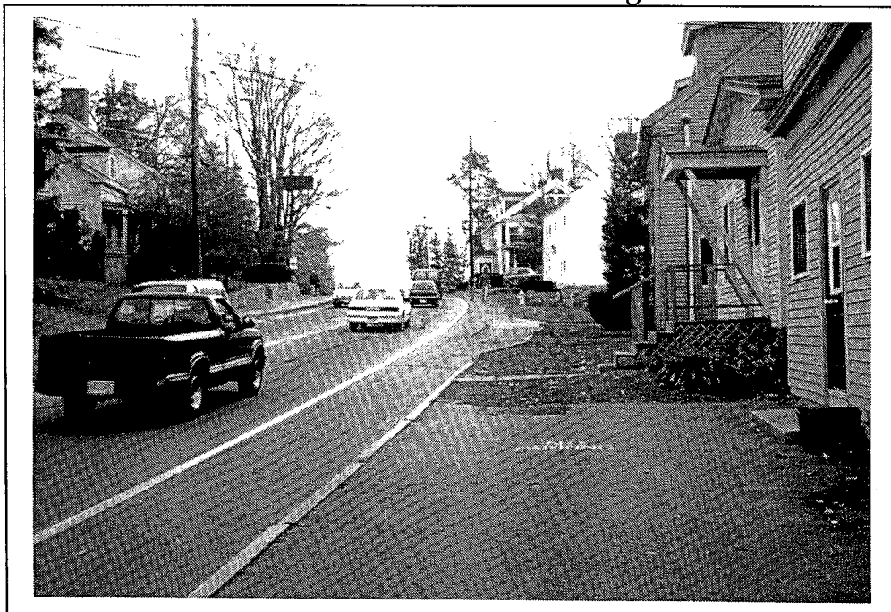
Existing conditions on Church Hill
