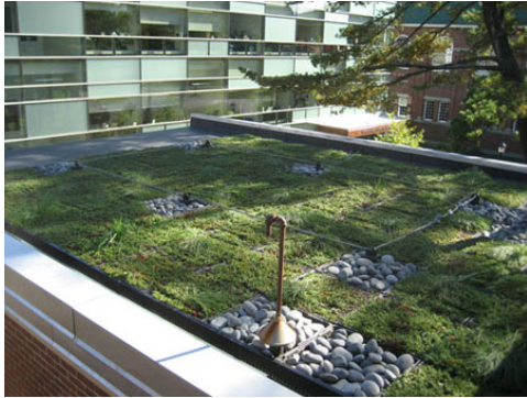
Newly installed green roof at Bowdoin College, Brunswick, ME (Image Credit: Richard Renner)
