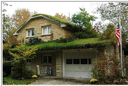
American green roof, Oswego, Illinois (Image Credit: Greg Robbins FLICKR)
