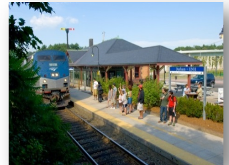
Photo 9: Rail Station - Downeaster (Photo Credit: UNH Photographic Services)
