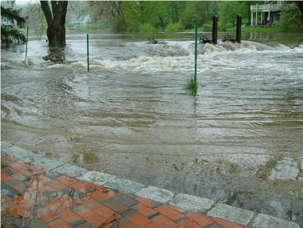
Oyster River Dam by Mill Pond, May 2006 Flood Event
