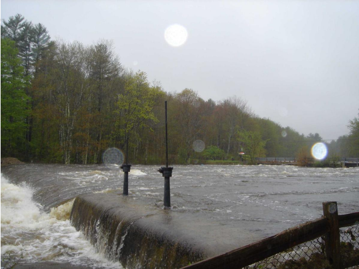
Wiswall Dam, May 2006 Flood
